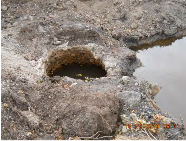
Figure 36 – Upstream manhole 08-100 US1 removed during reconstruction (major damage)
