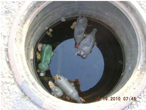
Figure 22 – Moderate floatables in catchbasin 16-201 US1
