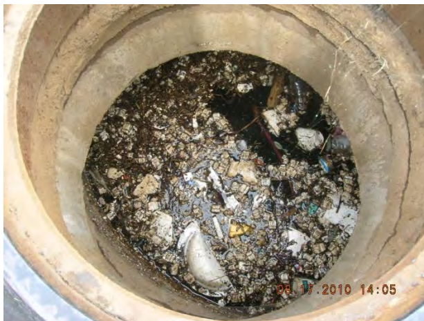
Figure 7 – Moderate floatables in manhole 03-173 US2
