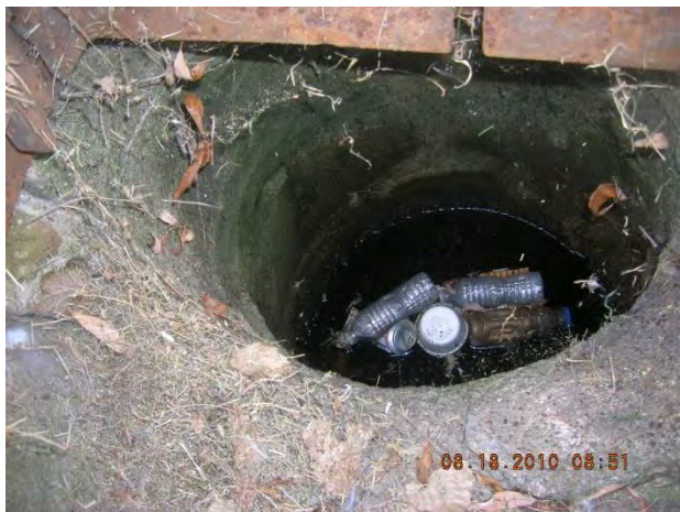
Figure 10 – Moderate floatables in curb inlet 03-381 US1
