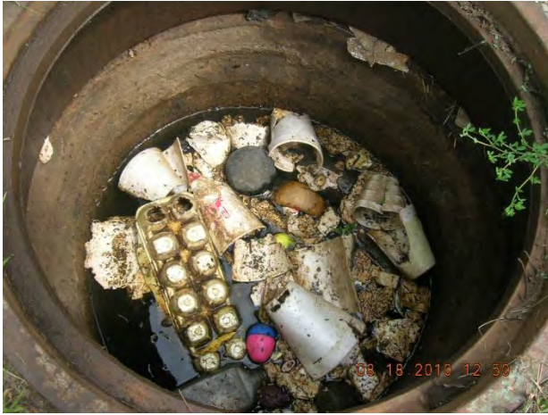
Figure 15 – Severe floatables in manhole 06-52 US1
