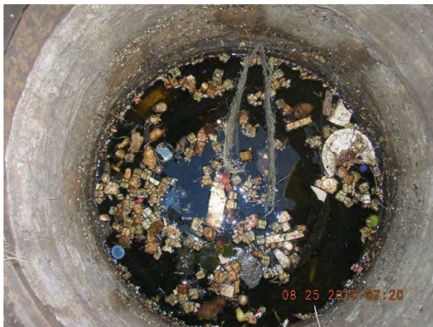
Figure 27 – Moderate floatables in manhole 16-551 US1
