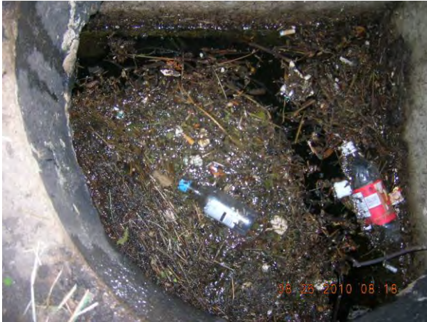
Figure 12 – Moderate floatables in manhole 05-264 US1
