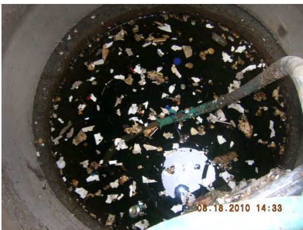
Figure 14 – Moderate floatables in manhole 06-221 US1
