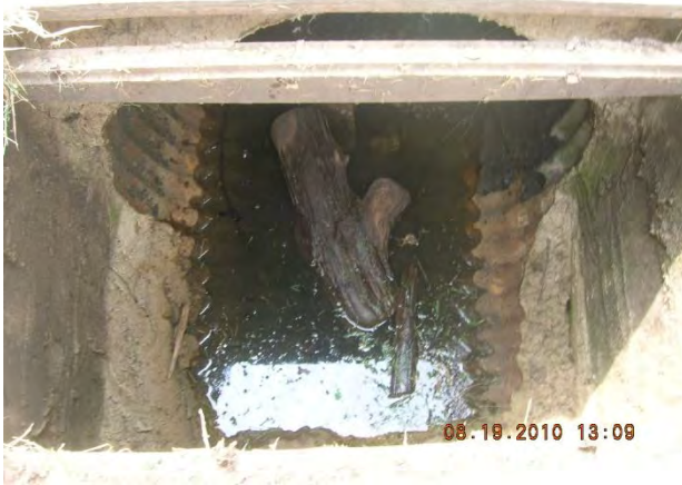
Figure 37 – Debris inside upstream catchbasin 12-890 US1 (minor damage)
