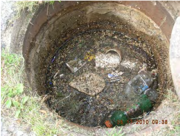
Figure 16 – Severe floatables in manhole 08-284 US1
