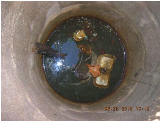
Figure 24 – Moderate floatables in manhole 16-436 US1
