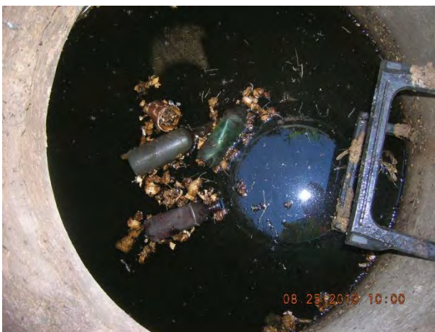
Figure 23 – Moderate floatables in manhole 16-396 US1
