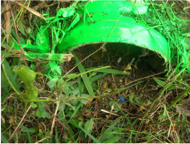
Figure 44 - Moderate deposition (3") at outfall 03-392
