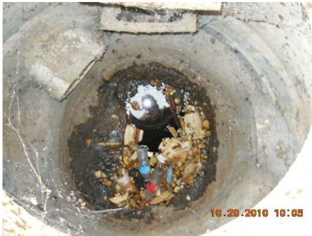
Figure 6 – Severe floatables in manhole 01-132 US1
