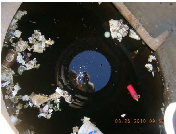
Figure 26 – Moderate floatables in manhole 16-533 US1
