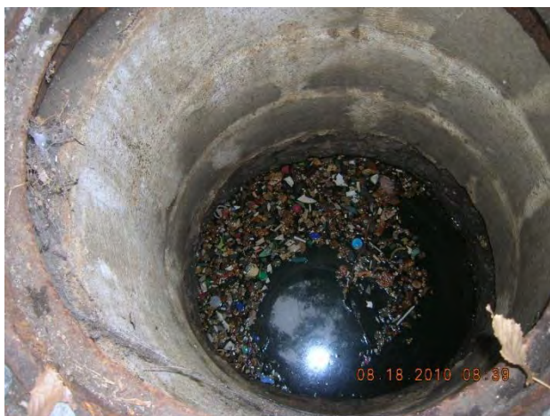
Figure 11 – Moderate floatables in manhole 03-81 US1
