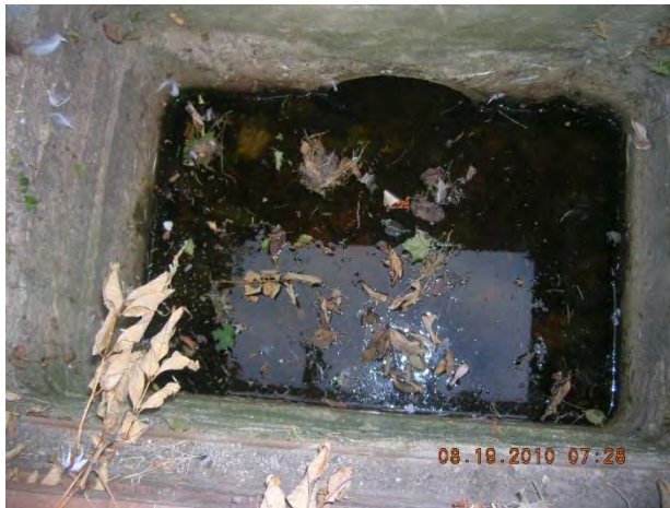
Figure 31 – Slight oil sheen in curb inlet 16-119 US1
