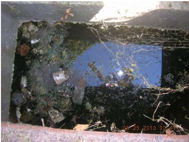
Figure 13 – Moderate floatables in curb inlet 06-1694 US1
