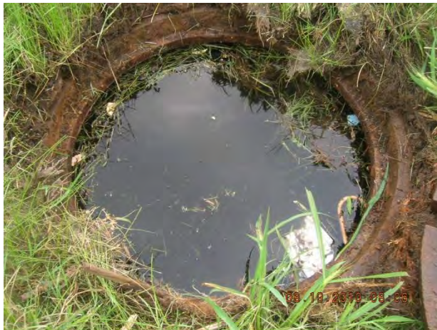
Figure 25 – Moderate floatables in manhole 16-463 US1
