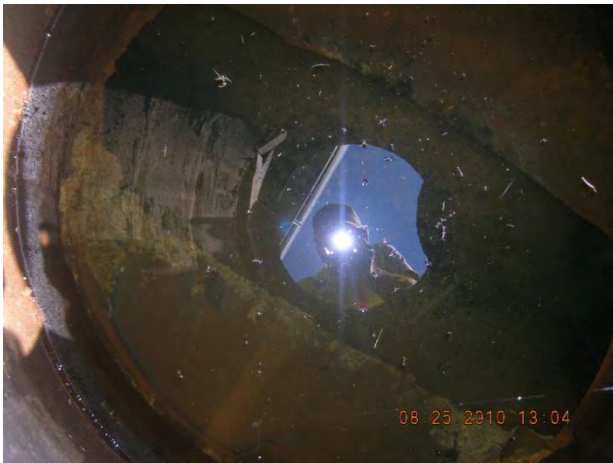
Figure 42 - Minor deposition (1") in manhole 01-360 US2
