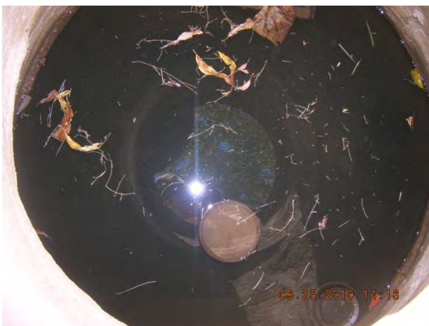
Figure 43 - Moderate deposition (12") in manhole 01-380 US1
