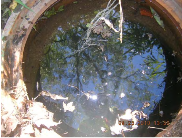
Figure 41 - Moderate deposition (4") in catchbasin 01-318 US1
