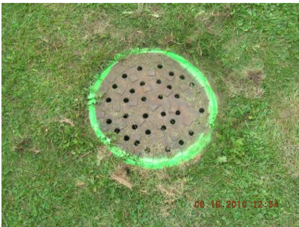
Figure 38 – Stuck lid at upstream manhole 12-972 US1
