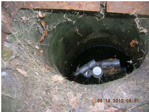
Figure 29 – Slight oil sheen in curb inlet 03-381 US1
