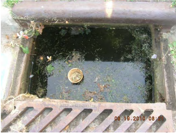
Figure 21 – Moderate floatables in curb inlet 16-142 US1
