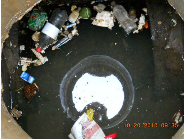
Figure 18 – Moderate floatables in manhole 09-101c US1
