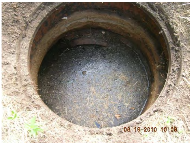
Figure 48 - Minor deposition (1") in manhole 16-362 US1
