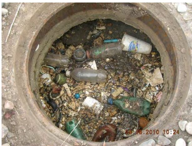
Figure 8 – Severe floatables in catchbasin 03-22 US1
