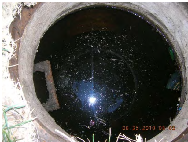
Figure 47 - Minor deposition (3") in manhole 16-164 US1
