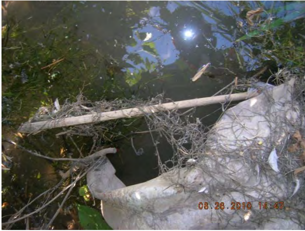
Figure 39 – Corrosion and crushed CMP at outfall 15-1093 (minor damage)
