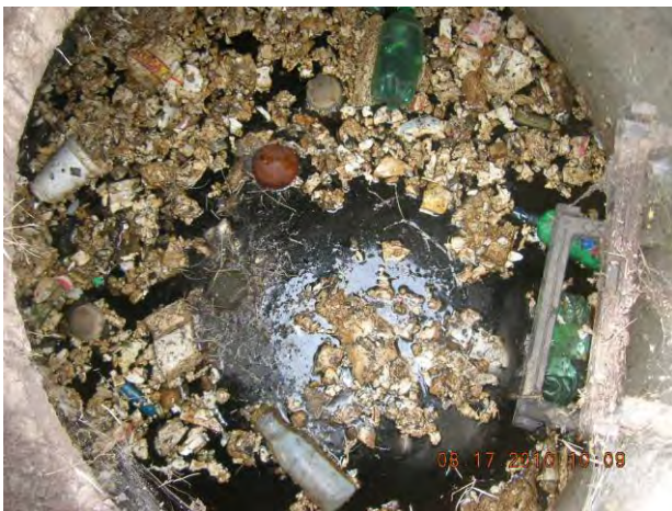
Figure 17 – Severe floatables in manhole 08-347 US1
