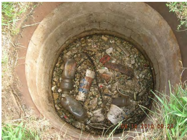
Figure 9 – Severe floatables in manhole 03-35 US1
