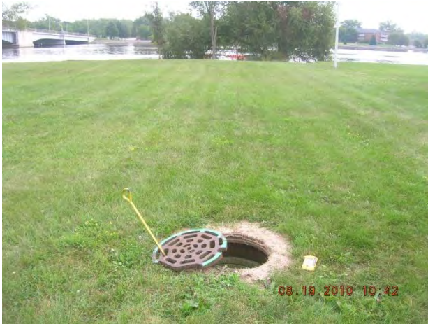
Figure 40 – Broken grate at upstream catchbasin 16-873 US1 (minor damage)
