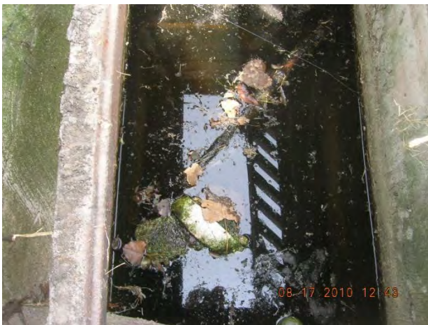
Figure 46 - Moderate deposition (8") in inlet 14-1075 US1
