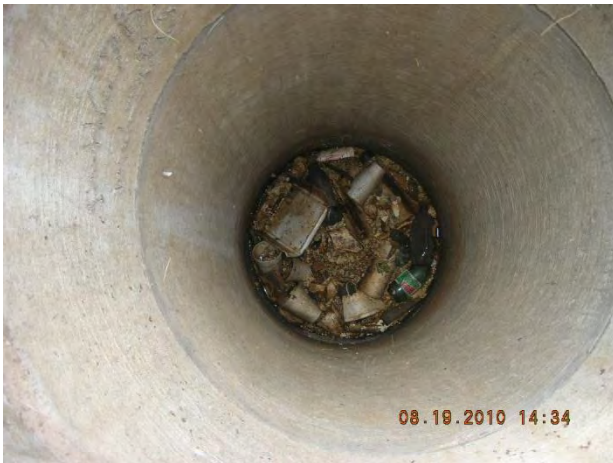
Figure 19 – Severe floatables in manhole 12-569 US1
