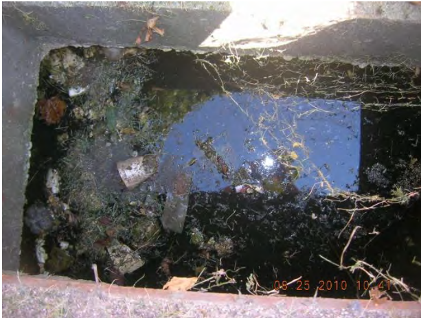
Figure 45 - Minor deposition (2") in inlet 06-1694 US1
