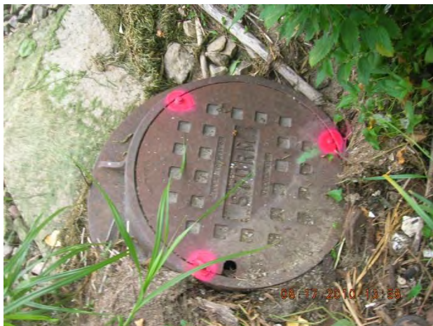
Figure 33 – Rusted/broken bolts at upstream manhole 03-173 US1 (moderate damage)
