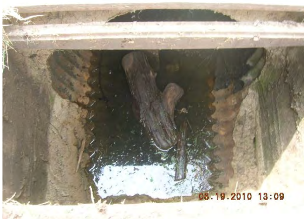
Figure 30 – Slight oil sheen in inlet 12-890 US1
