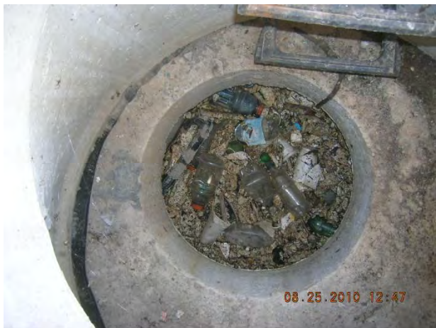
Figure 28 – Severe floatables in manhole 01-520 US1
