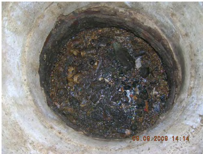
Figure 21 – Floatable debris and grease in upstream manhole 03-81 US1
