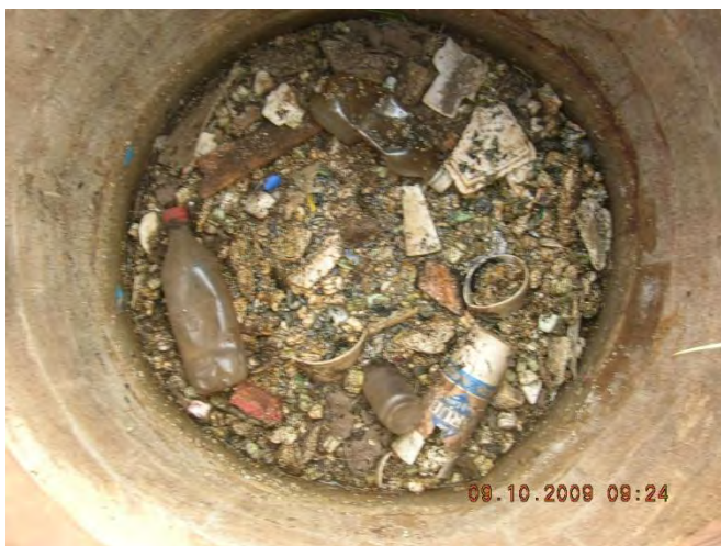
Figure 6 - Floatables in upstream manhole 03-35 US1
