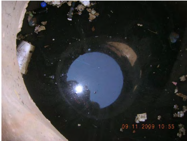
Figure 13 - Oil sheen in upstream manhole 09-101c US1
