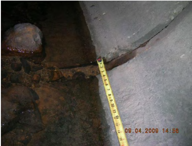
Figure 31 - Outfall 14-999 displaced pipe section
