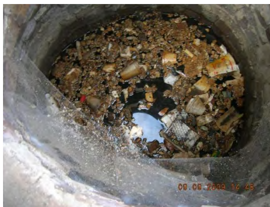
Figure 12 - Floatables in upstream manholes 03-81 US1 and US2 (with diesel fuel and grease)
