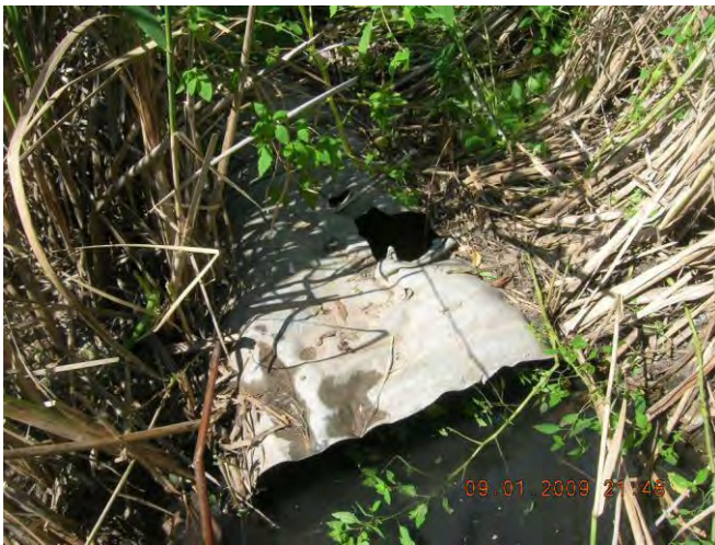
Figure 32 - Outfall 15-1067 crushed CMP with holes
