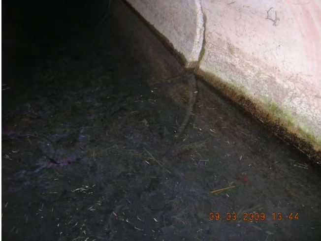
Figure 14 - Oil sheen in outfall 13-3099
