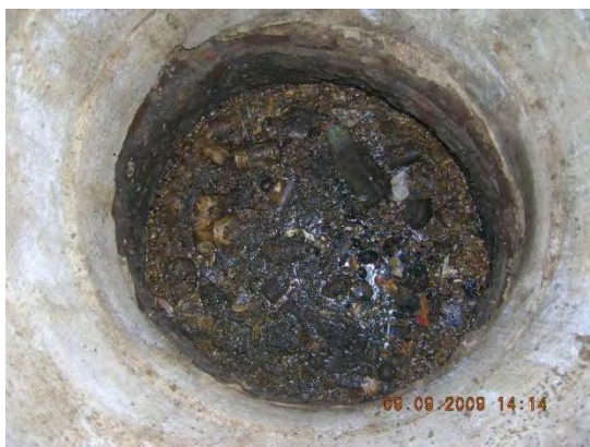
Figure 12 - Floatables in upstream manholes 03-81 US1 and US2 (with diesel fuel and grease)
