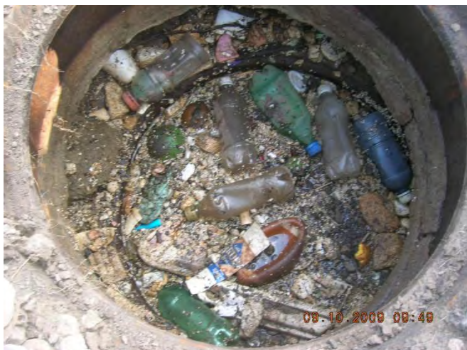
Figure 5 - Floatables in upstream manhole 03-22 US1
