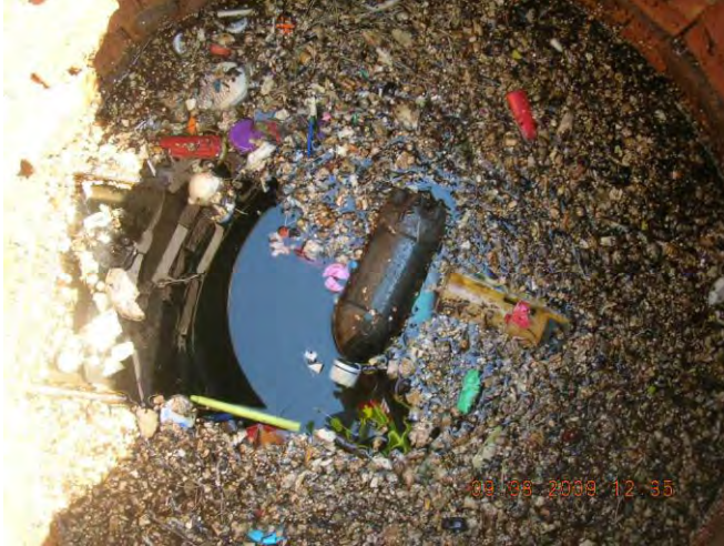
Figure 8 - Floatables in upstream manhole 11-376 US1
