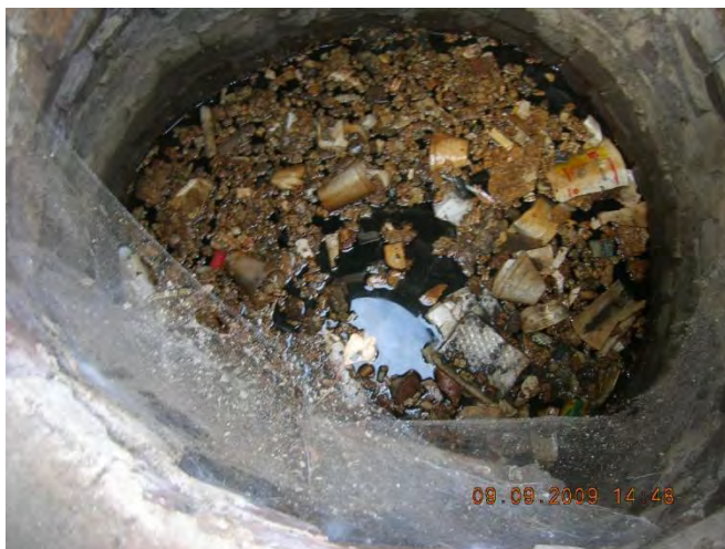
Figure 23 – Floatable debris in upstream manhole 03-81 US2
