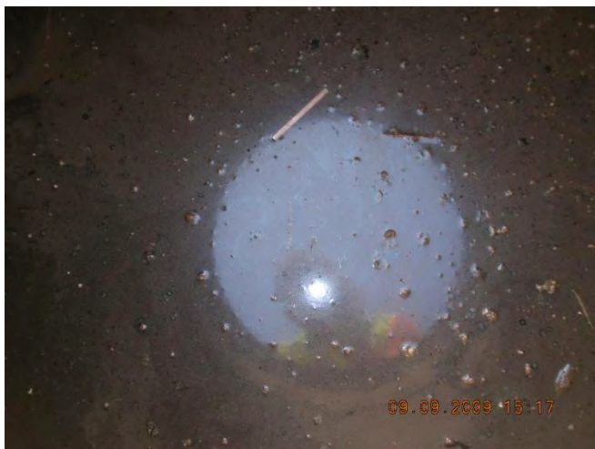
Figure 24 – Oil sheen in upstream manhole 03-81 US4
