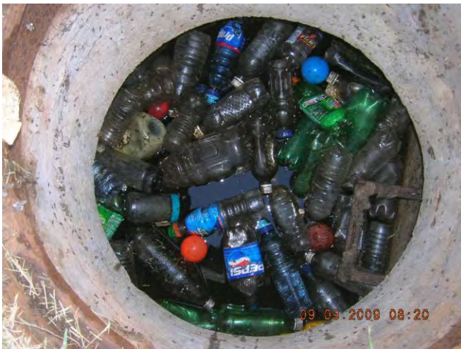
Figure 10 - Floatables in upstream manhole 12-576 US1
