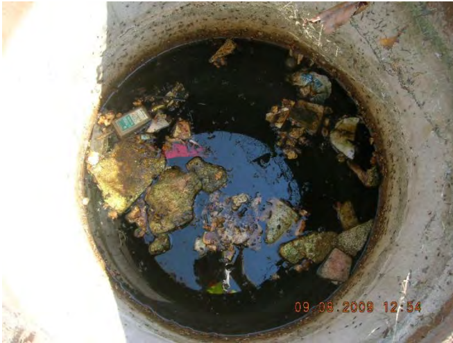
Figure 9 - Floatables in upstream manhole 11-465 US1
