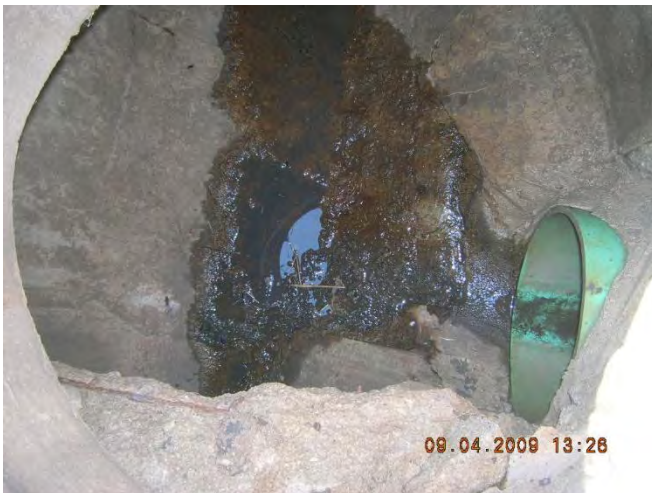
Figure 15 - Oil sheen in upstream manhole 14-595 US1
