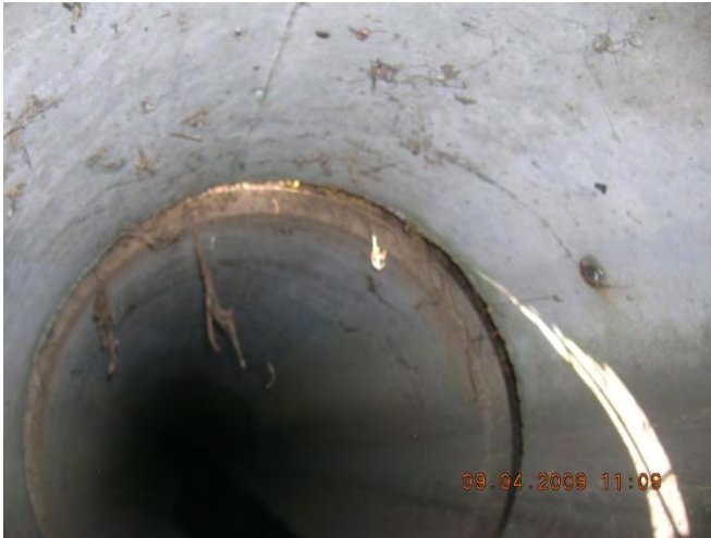
Figure 28 - Outfall 13-1554 displaced apron
