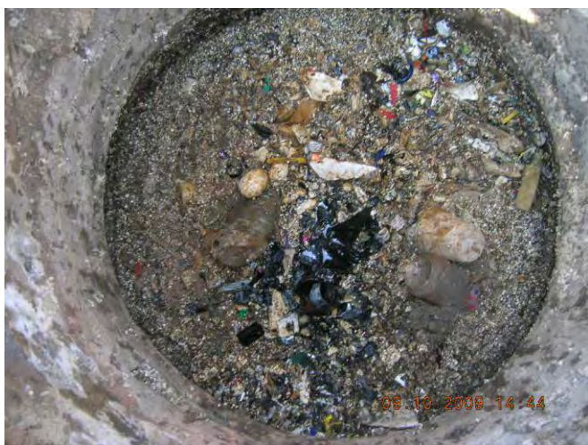
Figure 7 - Floatables in upstream manhole 06-560 US1
