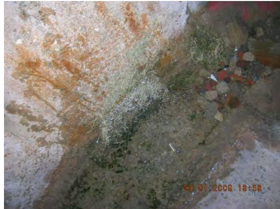
Figure 19 – Grass clippings in and around upstream manhole 15-1348 US2
