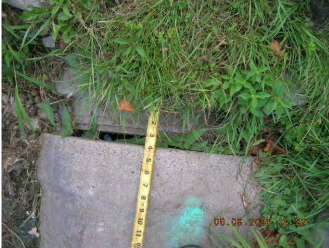
Figure 27 - Outfall 11-244 displaced pipe section
