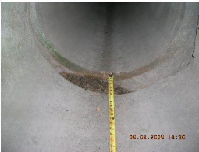
Figure 29 - Outfall 14-659 displaced apron
