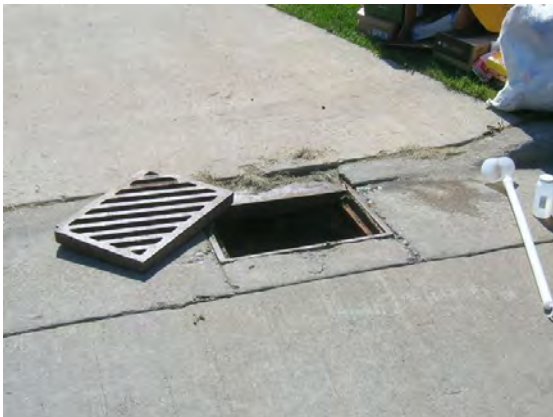
Figure 19 – Grass clippings in and around upstream manhole 15-1348 US2
