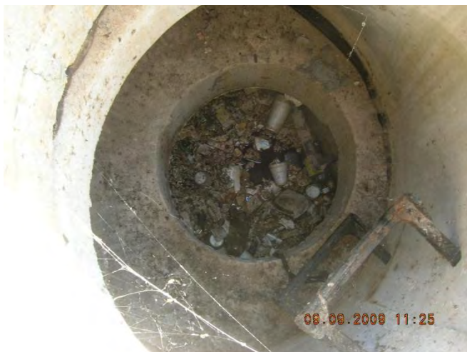
Figure 11 - Floatables in upstream manhole OSH-9424 US1
