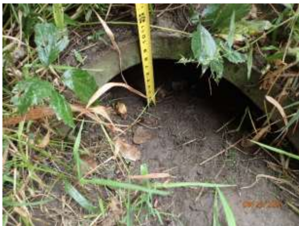
Figure 38 – Moderate deposition at outfall 13-3021
