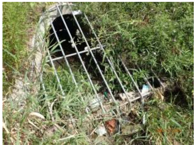
Figure 33 – Minor deposition at outfall 12-2551
