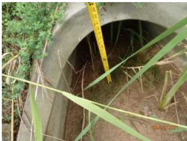
Figure 39 – Minor deposition at outfall 13-4107
