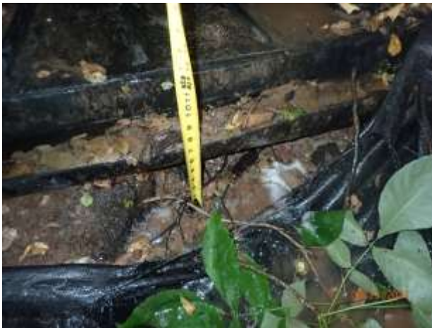
Figure 22 – Undercut apron at outfall 13-3130
