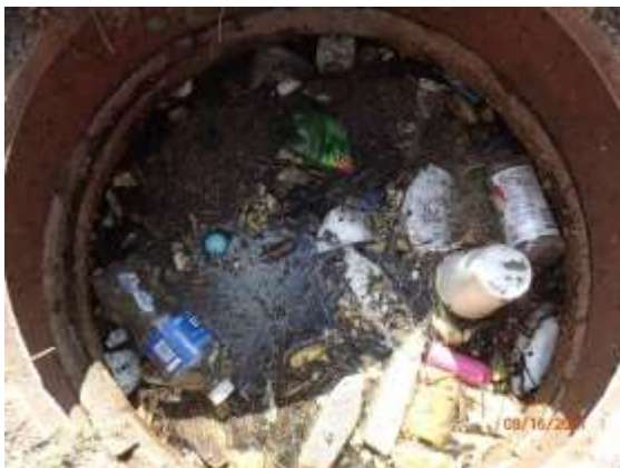
Figure 11 – Floating gross solids in manhole 05-14 US1
