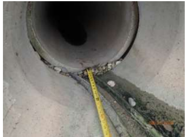
Figure 23 – Displaced apron at outfall 13-3636
