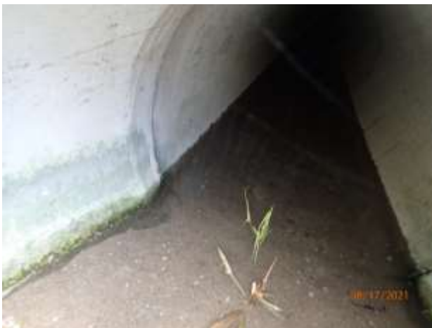
Figure 32 – Minor deposition at outfall 12-2538
