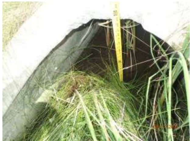
Figure 31 – Minor deposition at outfall 12-2128
