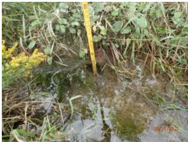
Figure 35 – Moderate deposition at outfall 13-1098
