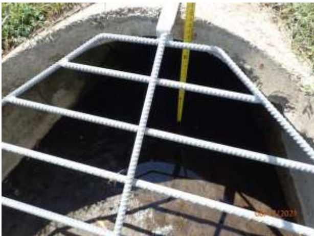
Figure 44 – Minor deposition at outfall 15-571
