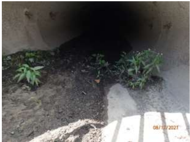
Figure 43 – Minor deposition at outfall 15-2412
