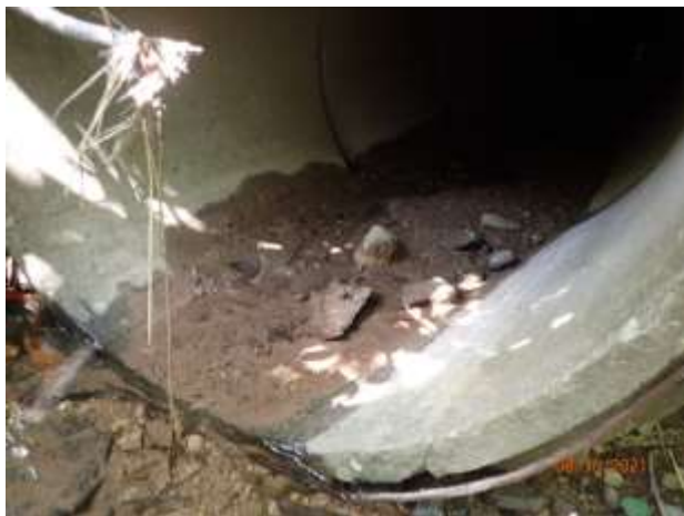
Figure 26 – Displaced pipe at outfall 14-999
