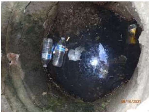
Figure 34 – Minor deposition in manhole 03-381 US1
