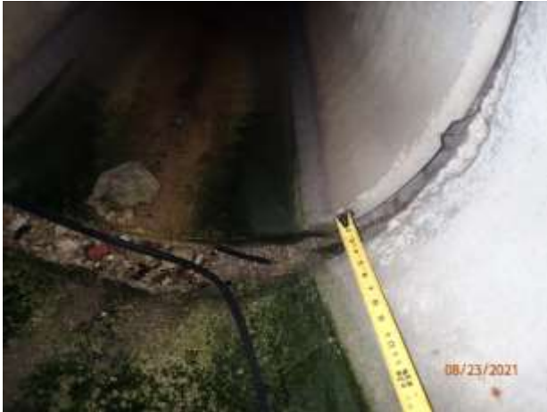
Figure 20 – Displaced apron at outfall 13-1673
