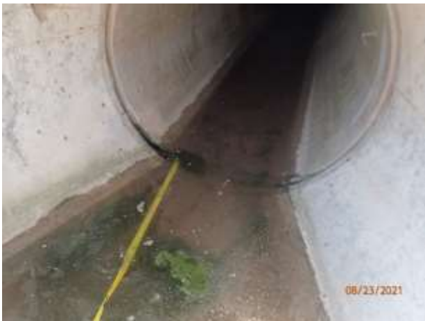
Figure 24 – Displaced apron at outfall 13-3861
