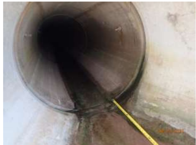
Figure 25 – Displaced apron at outfall 13-3869
