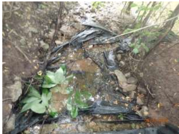
Figure 47 – Erosion downstream of outfall 13-3130
