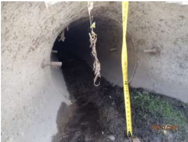
Figure 42 – Minor deposition at outfall 15-2409
