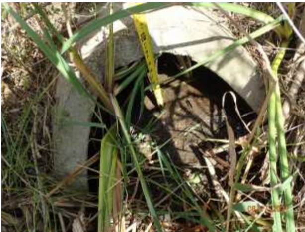
Figure 30 – Moderate deposition at outfall 12-2126
