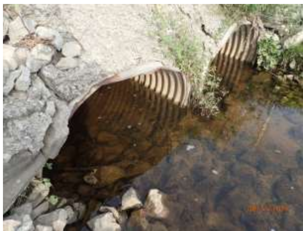
Figure 29 – Corrosion at outfall Wash41_03
