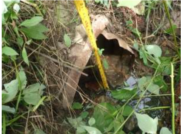
Figure 41 – Minor deposition at outfall 15-1217
