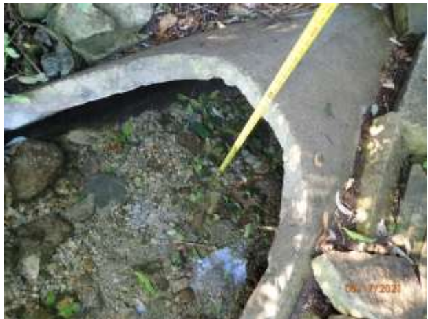
Figure 45 – Minor deposition at outfall 16-660
