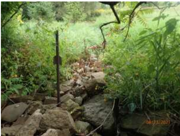
Figure 46 – Erosion downstream of outfall 13-2135
