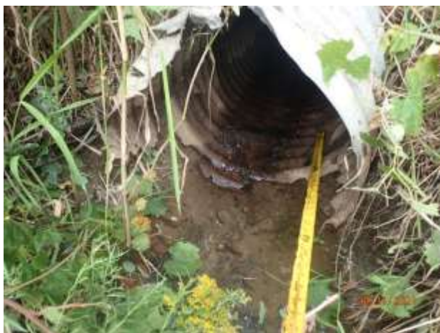
Figure 28 – Corrosion and crushing at outfall 15-1219
