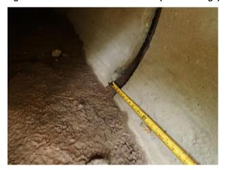
Figure 23 - Displacement at outfall 14-999 (minor damage)
