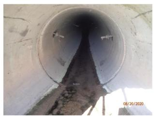
Figure 45 – Minor deposition at outfall 13-3706
