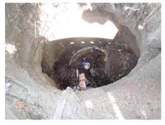
Figure 25 – Severe deposition in inlet 03-381 US1
