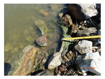
Figure 30 - Moderate deposition at outfall 09-32
