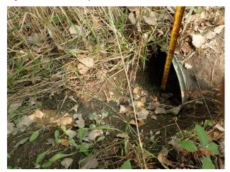
Figure 41 – Severe deposition at outfall 2464
