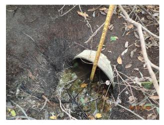
Figure 49 - Moderate deposition at outfall 15-2375
