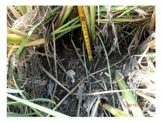
Figure 42 - Moderate deposition at outfall 13-2527
