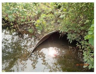
Figure 19 – Corrosion at outfall 13-1283 (minor damage)
