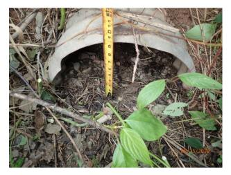
Figure 48 - Moderate deposition at outfall 15-1734
