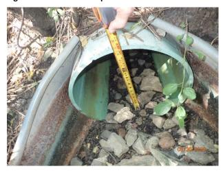
Figure 39 - Minor deposition at outfall 13-1870
