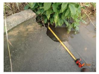
Figure 20 – Damaged concrete apron at outfall 13-2563 (minor damage)
