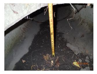
Figure 31 - Minor deposition at outfall 12-2042
