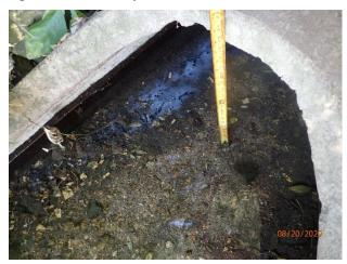
Figure 53 – Minor deposition at outfall 16-660
