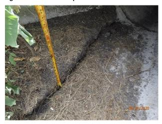
Figure 51 – Minor deposition at outfall 15-573
