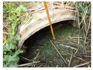
Figure 35 – Moderate deposition at outfall 13-1552
