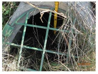
Figure 52 – Minor deposition at outfall 16-1205
