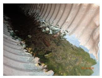
Figure 18 – Corrosion at outfall 13-1106 (severe damage)
