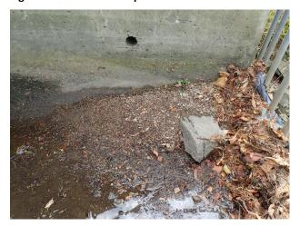
Figure 32 – Minor deposition at outfall 12-2273
