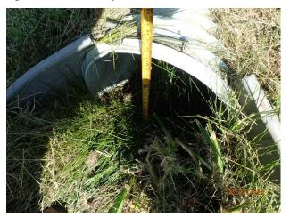
Figure 28 – Moderate deposition at outfall 06-154
