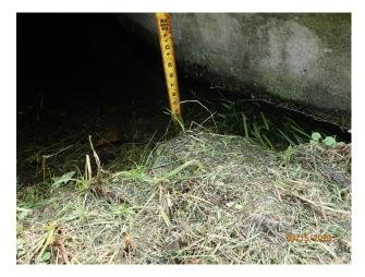
Figure 43 - Moderate deposition at outfall 13-2561
