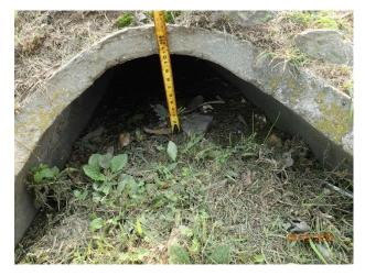
Figure 37 - Moderate deposition at outfall 13-1760
