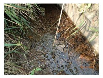
Figure 36 - Minor deposition at outfall 13-1758
