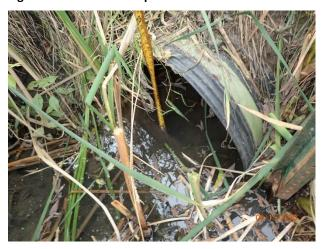
Figure 44 – Severe deposition at outfall 13-2564
