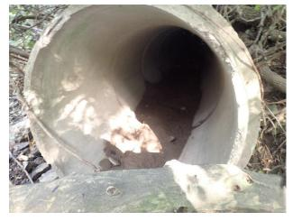
Figure 47 – Minor deposition at outfall 14-999
