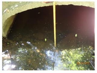
Figure 46 - Moderate deposition at outfall 13-471
