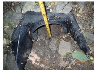
Figure 29 - Moderate deposition at outfall 06-1633
