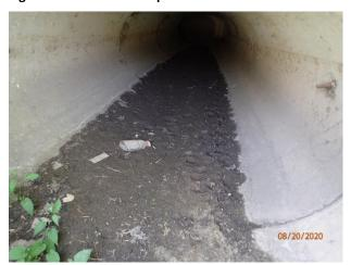
Figure 50 - Minor deposition at outfall 15-2412
