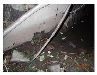
Figure 22 - Corrosion at outfall 13-68 (minor damage)
