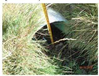
Figure 27 – Minor deposition at outfall 06-1161
