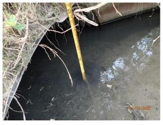
Figure 34 - Moderate deposition at outfall 13-1283
