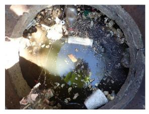
Figure 11 - Floating gross solids in manhole 03-22 US1
