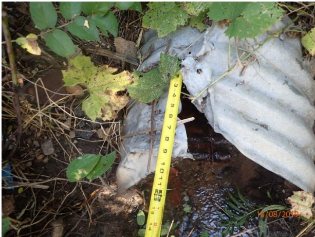
Figure 50 – Corrosion and damaged CMP at outfall 15-1219 (moderate damage)
