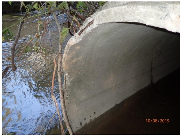
Figure 49 – Damaged end of pipe at outfall 14-999 (minor damage)
