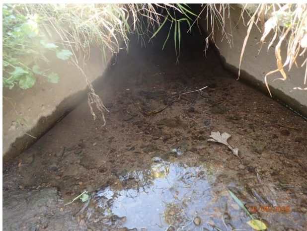
Figure 57 – Minor deposition at outfall 13-1758
