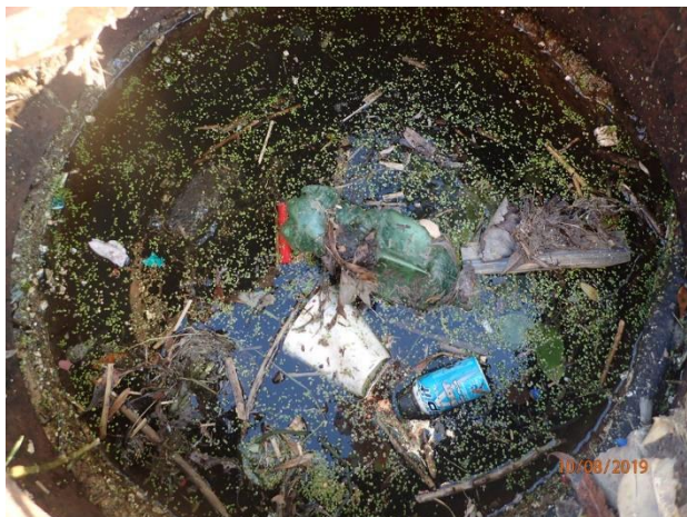
Figure 53 – Minor deposition in manhole 03-173 US1
