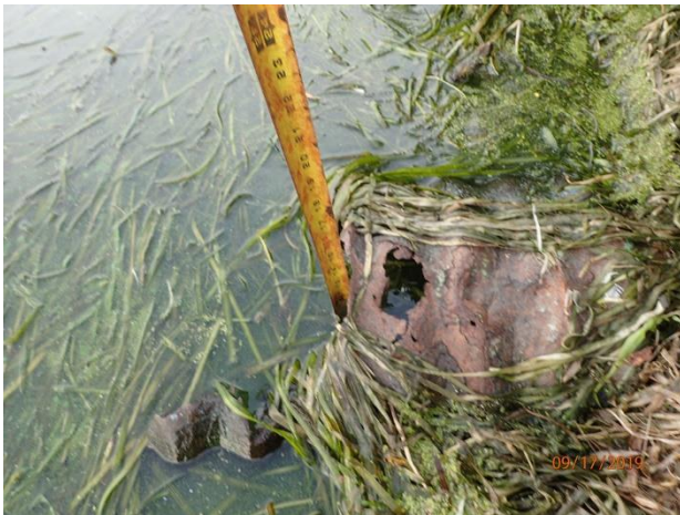
Figure 61 – Minor deposition at outfall 15-690
