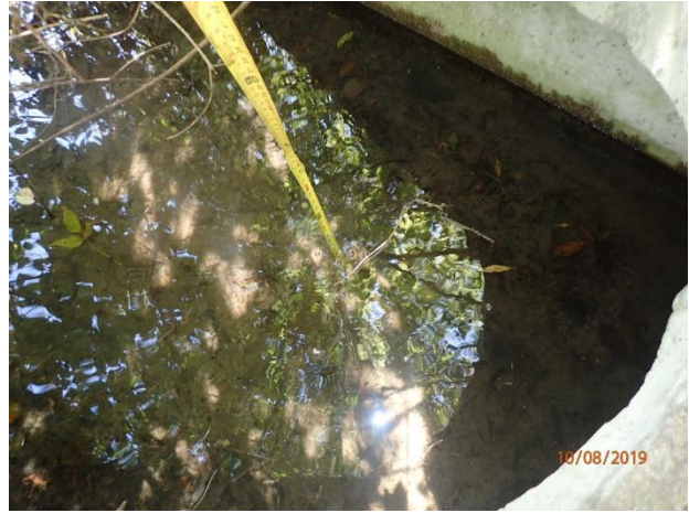
Figure 60 – Minor deposition at outfall 15-2108
