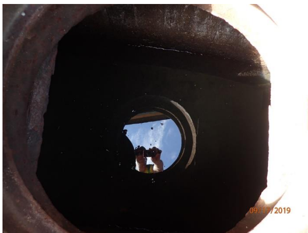
Figure 55 – Minor deposition in manhole 11-225 US2
