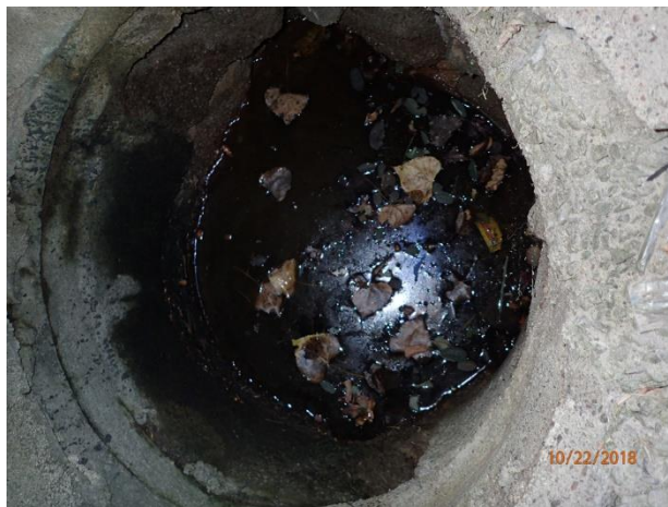
Figure 54 – Moderate deposition in manhole 03-381 US1
