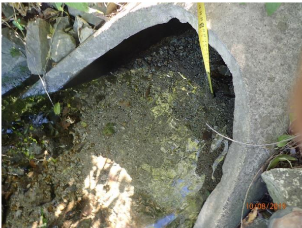
Figure 63 – Minor deposition at outfall 16-660
