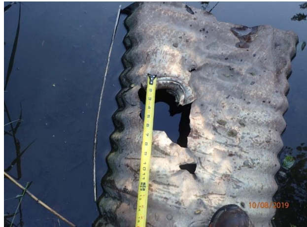
Figure 51 – Damaged CMP at outfall 15-1067 (moderate damage)
