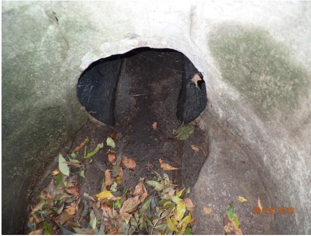
Figure 59 – Minor deposition in manhole 15-1137 US1
