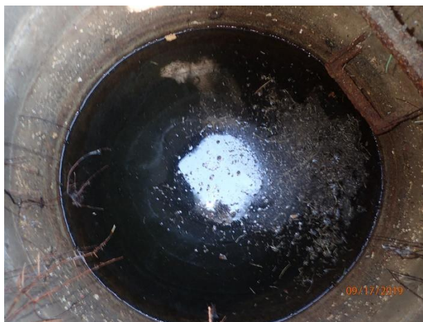
Figure 56 – Moderate deposition in manhole 11-71 US1
