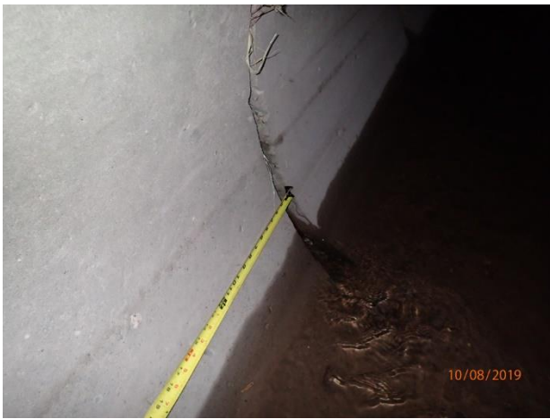
Figure 48 – Joint displacement at outfall 14-999 (minor damage)
