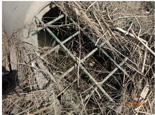
Figure 62 – Minor deposition at outfall 16-1205
