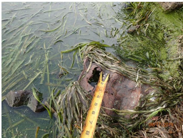
Figure 52 – Damaged CMP at outfall 15-690 (moderate damage)
