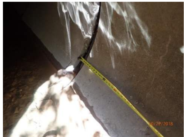
Figure 39 – Joint displacement at outfall 14-999 (moderate damage)
