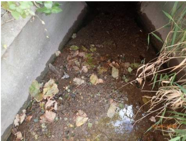
Figure 40 – Minor deposition at outfall 13-1588
