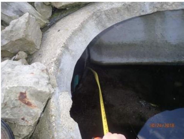
Figure 38 – Apron displacement at outfall 13-2872a (minor damage)
