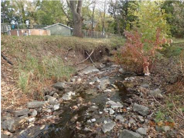
Figure 49 – Bank erosion downstream of outfall 13-471
