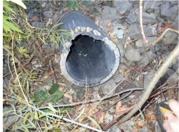
Figure 37 – Damaged end of pipe at outfall 13-1109 (minor damage)
