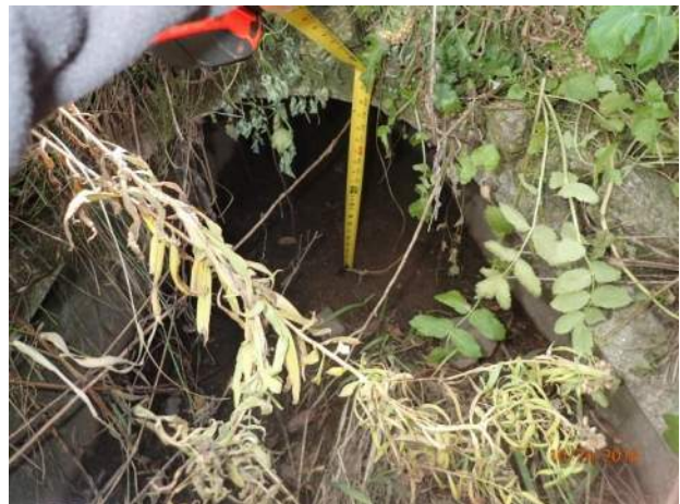
Figure 43 – Minor deposition at outfall 13-2867
