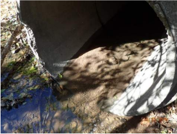
Figure 44 – Minor deposition at outfall 14-999
