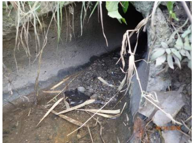
Figure 41 – Minor deposition at outfall 13-2611
