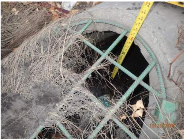
Figure 48 – Minor deposition at outfall 16-1205
