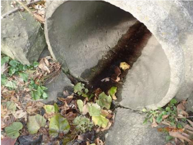
Figure 36 – Joint displacement at outfall 06-478 (minor damage)
