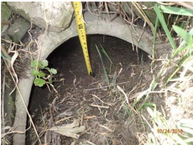
Figure 42 – Moderate deposition at outfall 13-2860
