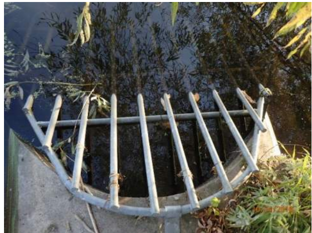
Figure 47 – Minor deposition at outfall 15-2477
