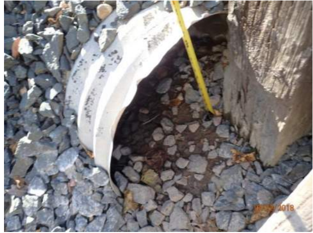
Figure 45 – Moderate deposition at outfall 14-1514
