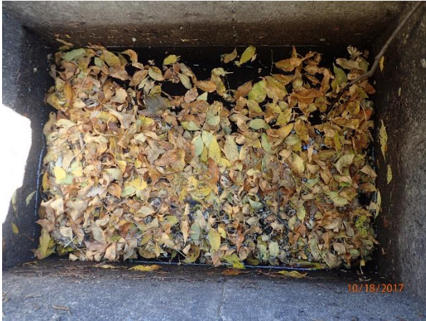
Figure 54 – Moderate deposition in inlet 06-1028 US1
