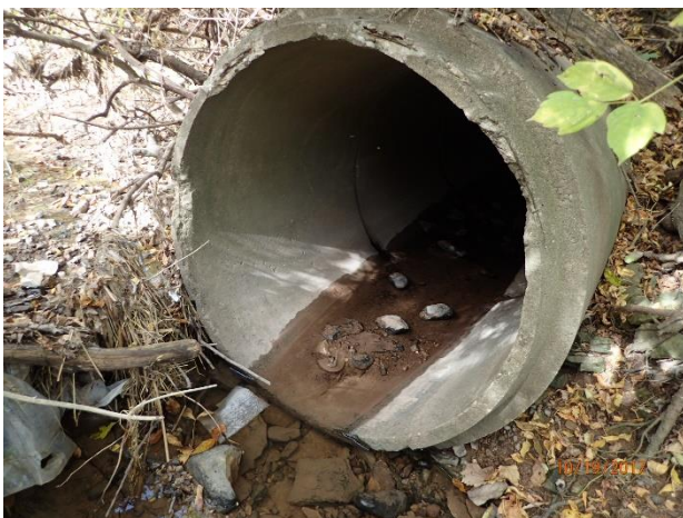
Figure 46 – Damaged concrete at outfall 14-999 (minor damage)
