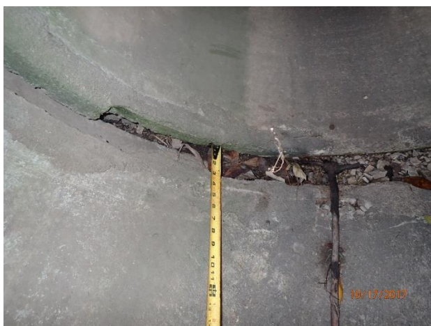
Figure 40 – Apron displacement at outfall 06-1132 (moderate damage)
