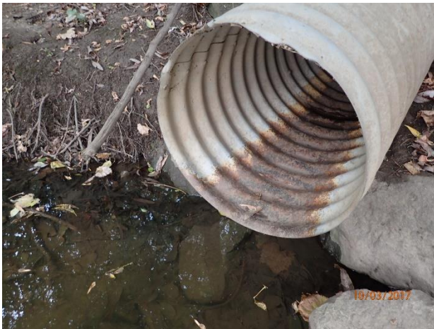
Figure 50 – Corrosion at outfall 16-629 (minor damage)
