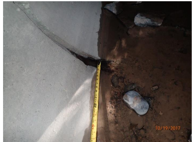
Figure 45 – Apron displacement at outfall 14-999 (moderate damage)
