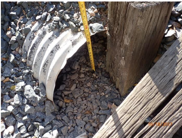
Figure 64 – Moderate deposition at outfall 14-1514
