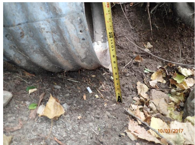
Figure 47 – Undercut pipe at outfall 16-622 (minor damage)
