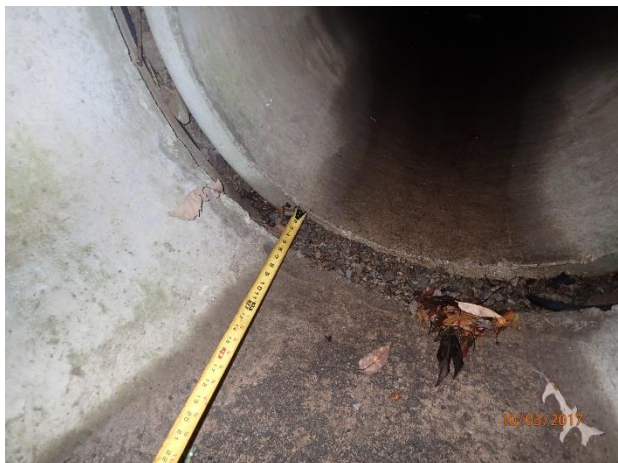
Figure 38 – Apron displacement at outfall 06-977 (moderate damage)
