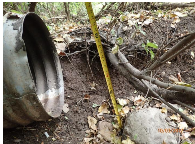
Figure 74 – Moderate erosion downstream of outfall 16-622
