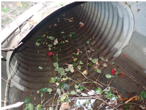
Figure 36 – Corrosion at outfall 06-3 (minor damage)
