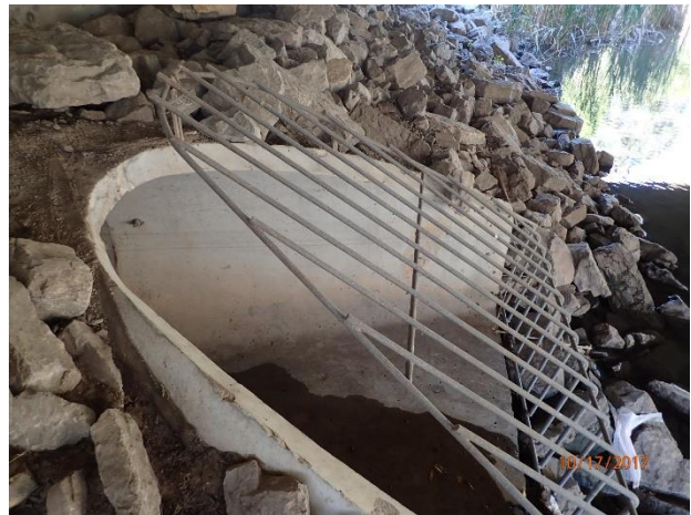
Figure 51 – Detached grate at outfall 16-646a (minor damage)
