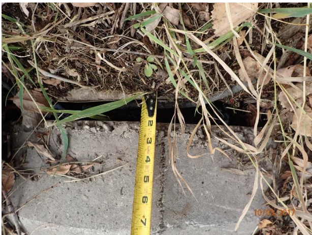
Figure 52 – Apron displacement at outfall 16-663 (moderate damage)
