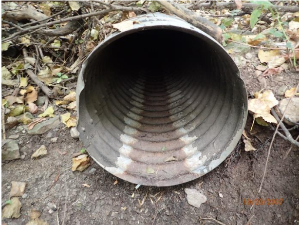
Figure 48 – Corrosion at outfall 16-622 (minor damage)
