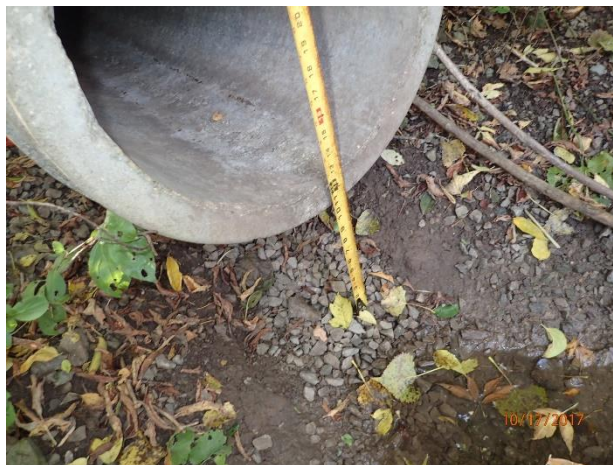
Figure 37 – Undercut pipe at outfall 06-961 (moderate damage)
