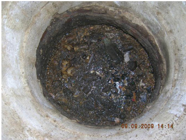
Figure 15 – Floatable debris and grease in upstream manhole 03-81 US1 (2009)
