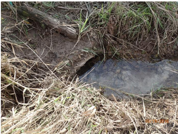
Figure 58 – Moderate deposition at outfall 13-1098
