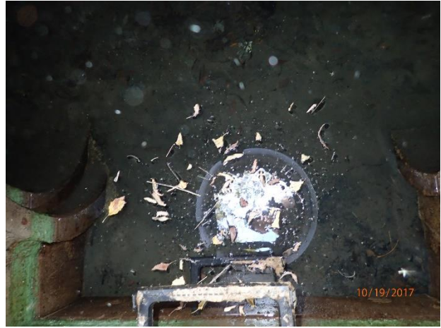
Figure 67 – Minor deposition in manhole 15-2477 US2
