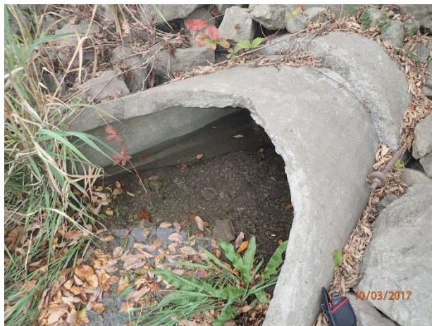
Figure 39 – Chipped concrete apron at outfall 06-1083 (minor damage)
