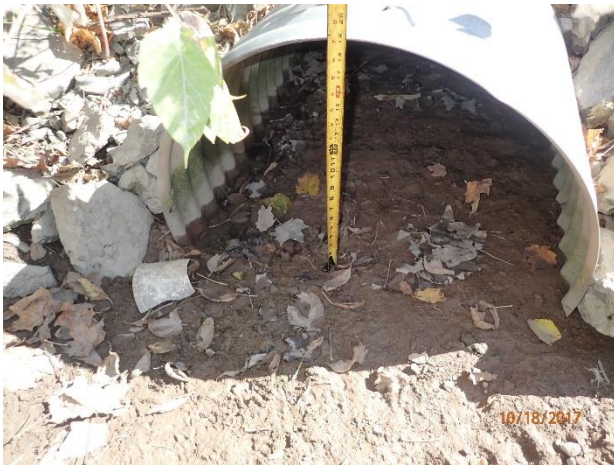
Figure 62 – Moderate deposition at outfall 14-766
