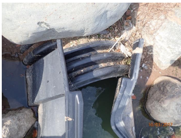
Figure 41 – Missing apron clamp at outfall 06-1495 (minor damage)
