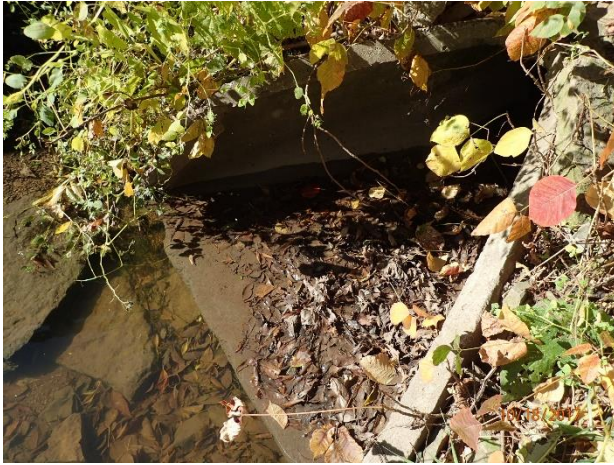
Figure 42 – Apron displacement at outfall 14-645 (minor damage)
