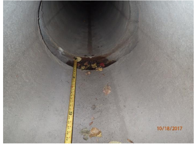
Figure 43 – Apron displacement at outfall 14-659 (moderate damage)
