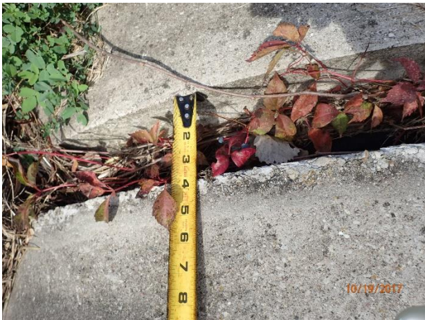
Figure 44 – Apron displacement at outfall 14-996 (moderate damage)
