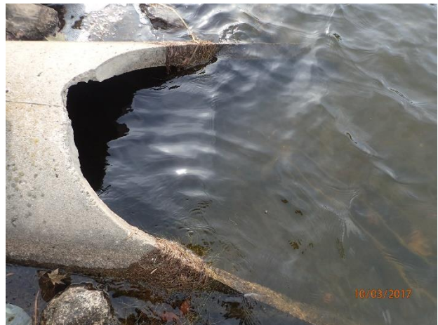
Figure 53 – Chipped concrete apron at outfall 16-941 (minor damage)
