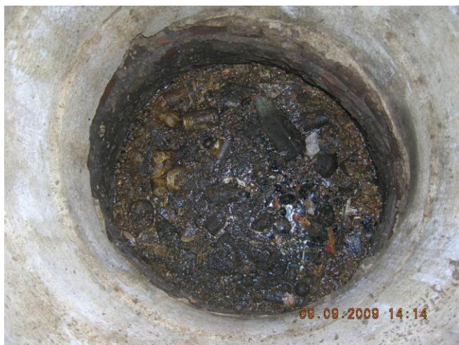
Figure 14 – Floatable debris and grease in upstream manhole 03-81 US1 (2009)
