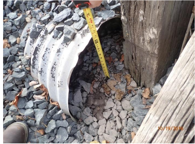
Figure 25 – Moderate deposition in outfall 14-1514
