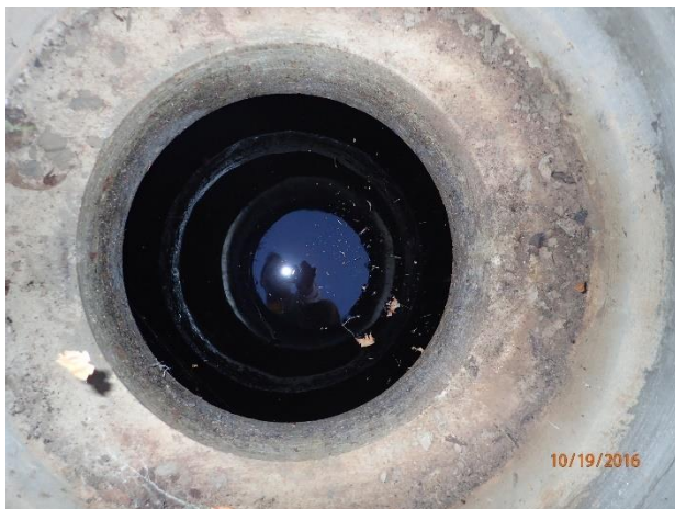
Figure 22 – Minor deposition in manhole 11-1097 US1
