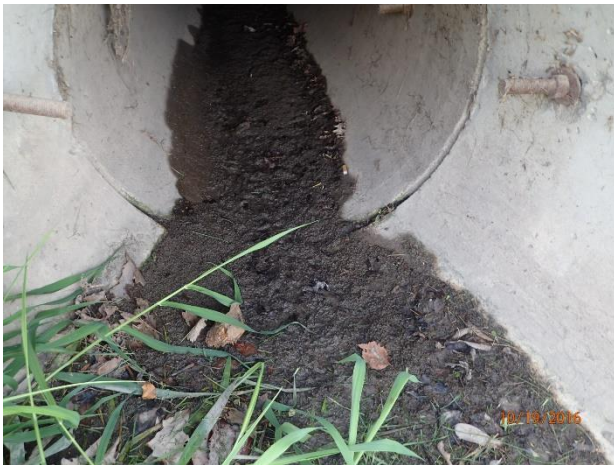
Figure 26 – Minor deposition at outfall 15-2409
