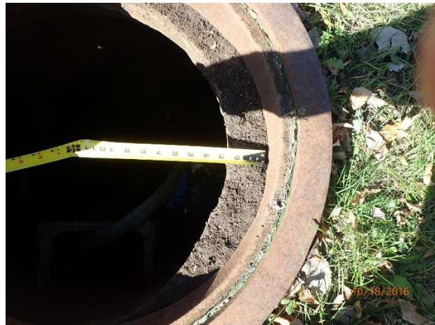
Figure 20 – Displaced casting at manhole 06-221 US1 (minor damage)
