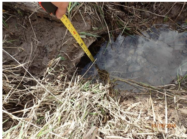
Figure 23 – Severe deposition at outfall 13-1098
