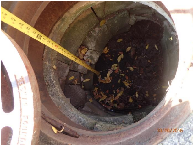
Figure 28 – Minor deposition at catchbasin 16-47 US2
