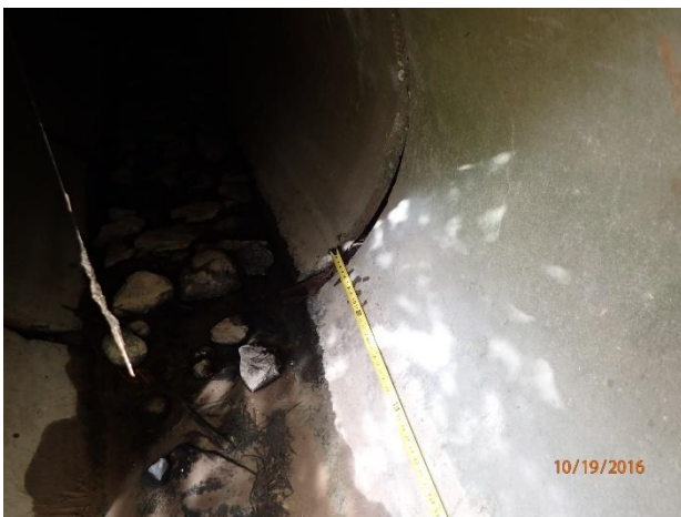
Figure 21 – 4" joint displacement at outfall 14-999 (minor damage)
