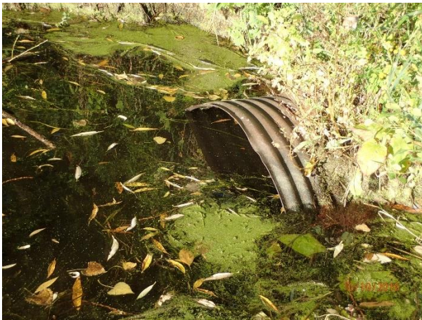
Figure 19 – Corrosion at outfall 03-293 (minor damage)
