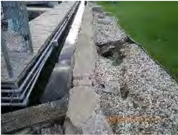
Figure 18 – Significant settling at outfall 03-22 (severe damage)
