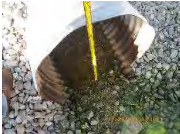
Figure 31 – Minor deposition at outfall 13-1106
