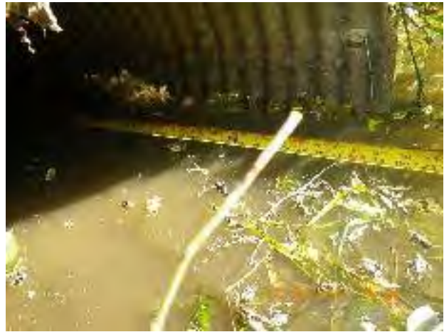
Figure 19 – Corroded metal pipe at outfall 12-890 (moderate damage)
