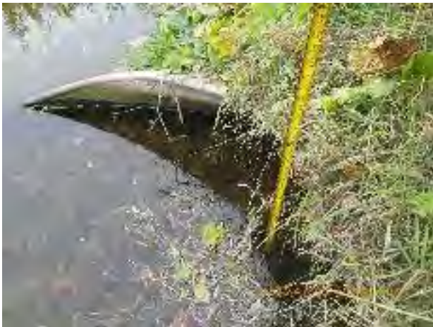
Figure 22 – Corroded metal pipe at outfall 13-1283 (minor damage)
