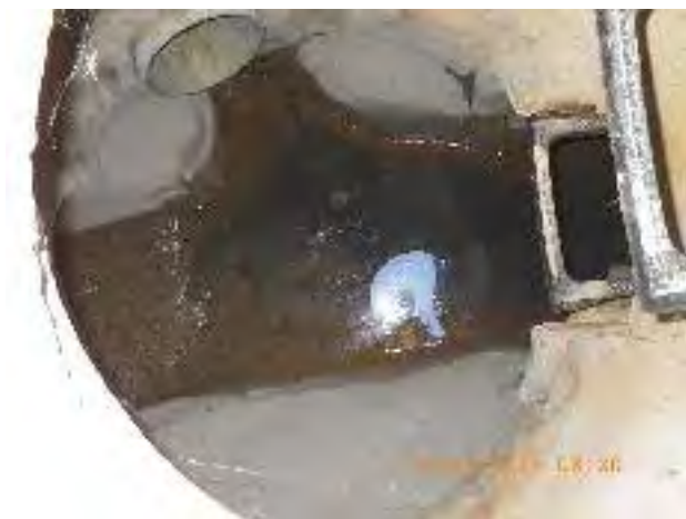
Figure 36 – Minor deposition in manhole 13-1769 US1
