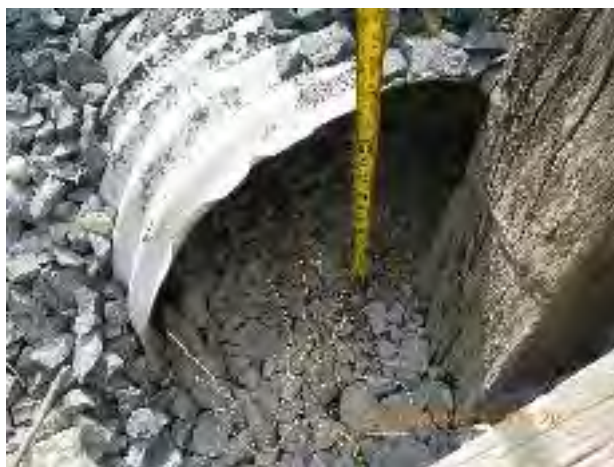
Figure 37 – Moderate deposition at outfall 14-1514
