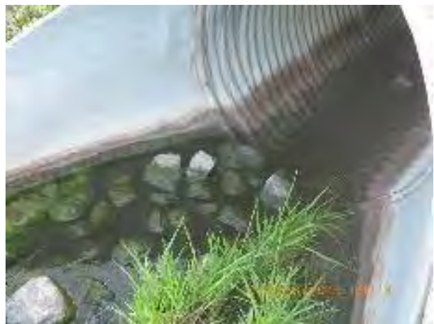
Figure 25 – Corroded metal pipe at outfall Wash41_01 US1 (minor damage)
