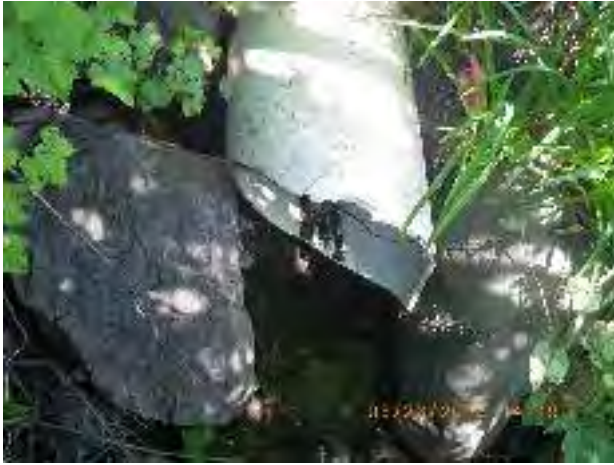
Figure 20 – Broken PVC pipe at outfall 12-972 (minor damage)
