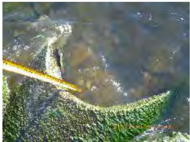
Figure 27 – Moderate deposition at outfall 02-105
