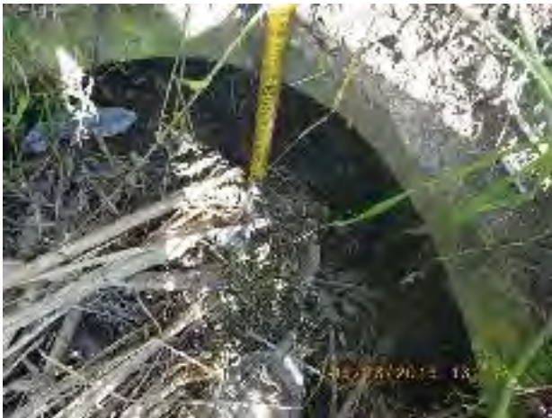
Figure 30 – Moderate deposition at outfall 12-2034
