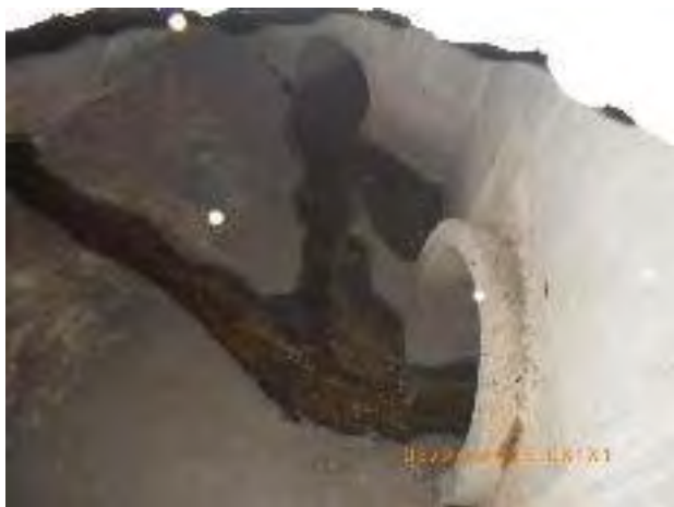
Figure 38 – Minor deposition in manhole 15-146 US1
