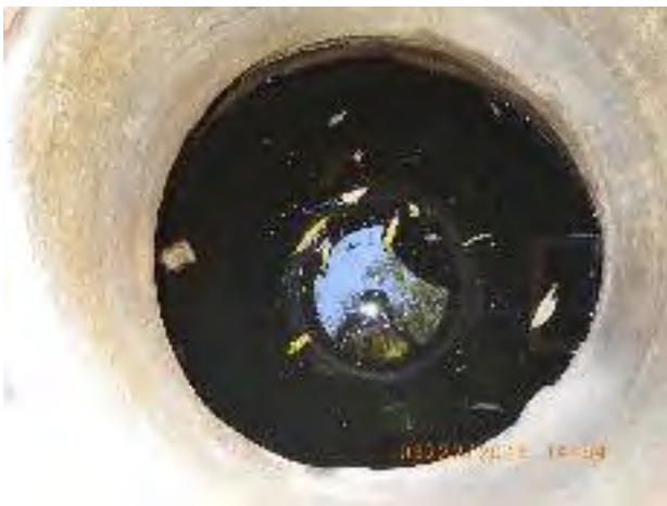
Figure 26 – Moderate deposition in manhole 01-380 US1
