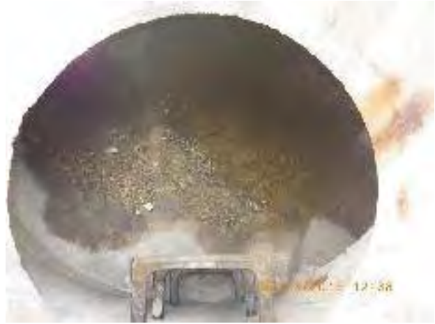
Figure 29 – Minor deposition in manhole 12-1795 US1
