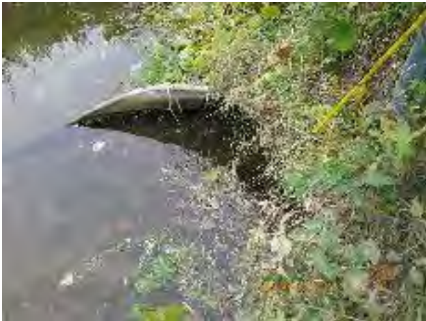
Figure 32 – Moderate deposition at outfall 13-1283
