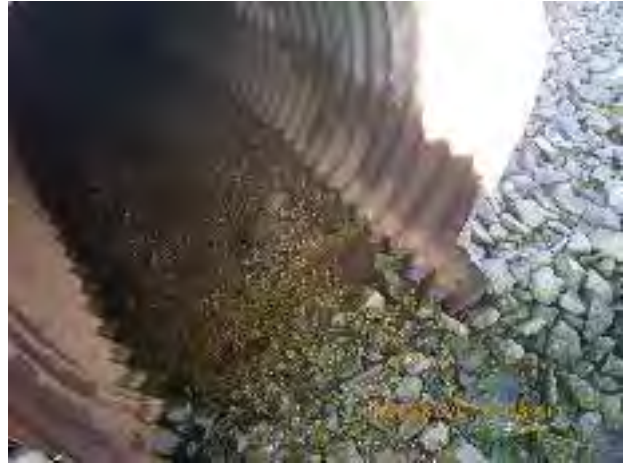
Figure 21 – Corrosion and crushed pipe at outfall 13-1106 (minor damage)
