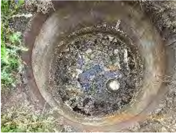
Figure 28 – Minor deposition in manhole 03-35 US1
