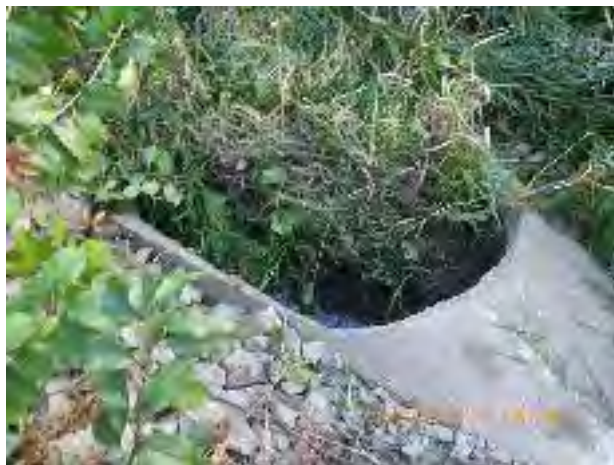
Figure 35 – Severe deposition at outfall 13-1769
