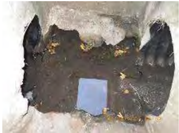
Figure 23 – Eroded flowline in manhole 13-68 US1 (minor damage)
