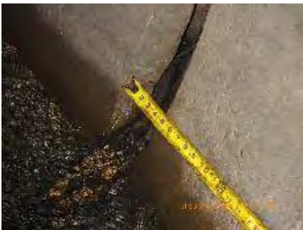
Figure 24 – 4" joint displacement at outfall 14-999 (moderate damage)
