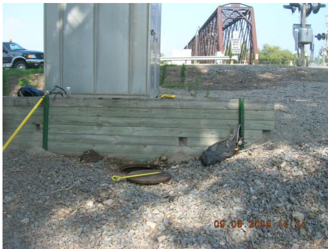
Figure 18 – Upstream manhole 03-81 US1 (2009)
