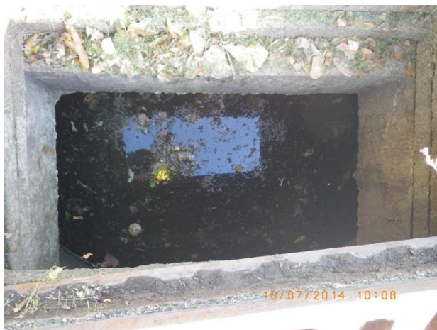
Figure 37 – Moderate deposition in inlet 06-1694 US1
