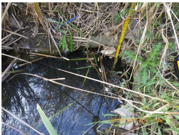
Figure 41 – Moderate deposition at outfall 13-1758
