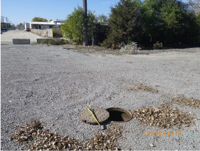
Figure 25 – Upstream manhole 03-81 US4 (2014)
