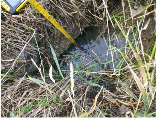
Figure 45 - Moderate deposition at outfall 13-2611
