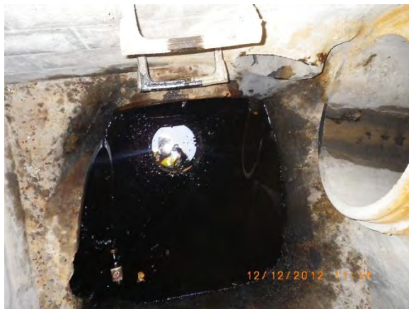
Figure 12 – Pipe from southwest branch entering manhole 13-1724 above the water level
