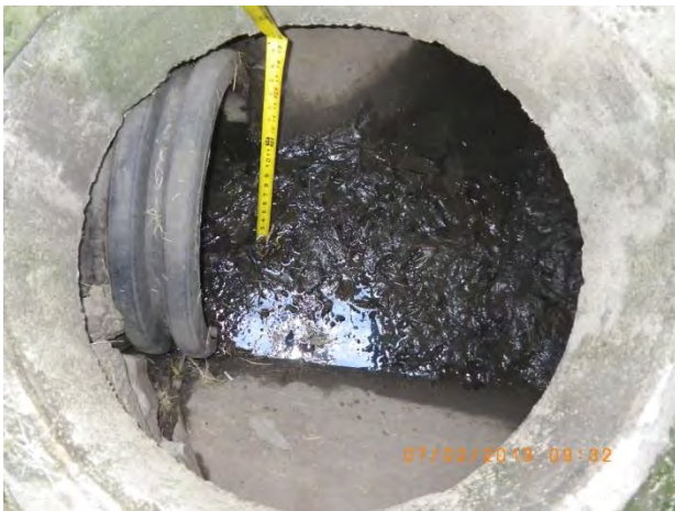
Figure 55 - Minor deposition at manhole 15-1702 US1
