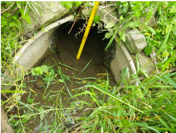
Figure 47 - Minor deposition at outfall 13-68
