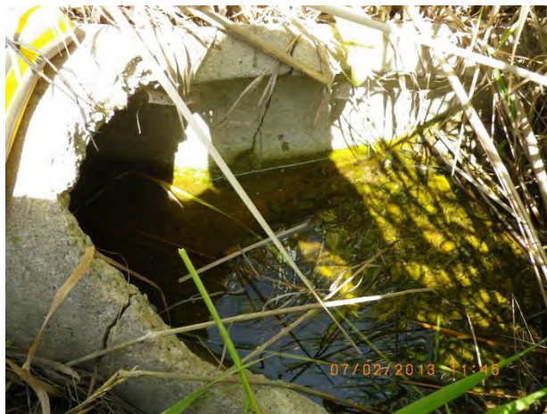
Figure 40 - Minor deposition at outfall 12-1916
