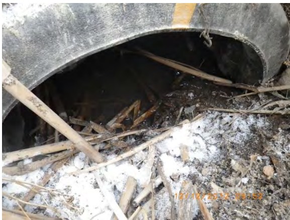
Figure 3 – Private storm sewer outfall in swale
