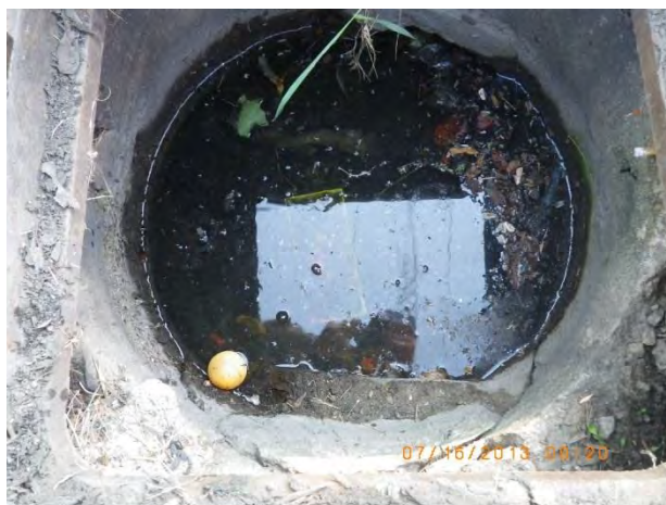
Figure 64 - Minor deposition at manhole 15-1891 US1
