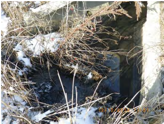
Figure 14 – Sheen on pool in upstream end of STH 44 culvert
