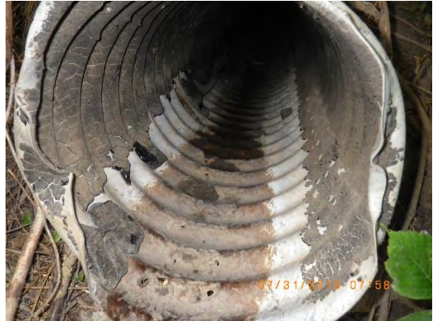
Figure 29 – Corrosion and undercutting at outfall 14-124 (moderate damage)
