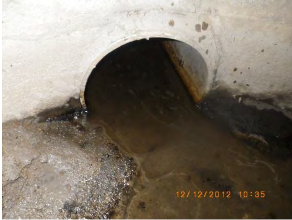
Figure 6 – Slight sheen in manhole 13-1749
