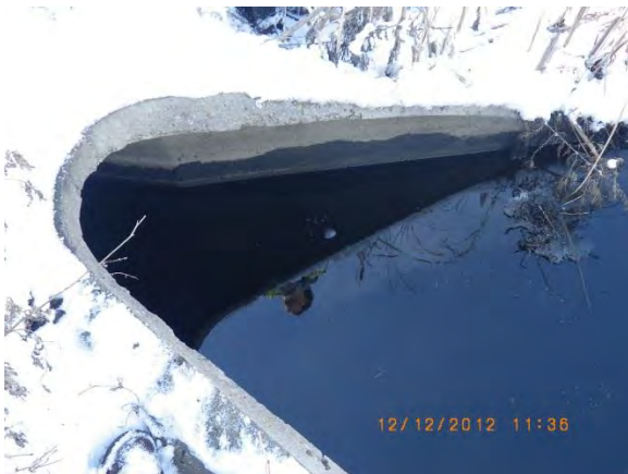
Figure 15 – Sheen on pool in downstream end of STH 44 culvert
