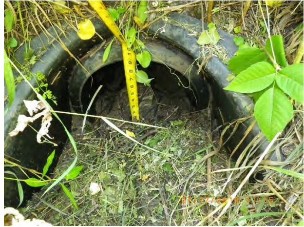
Figure 52 - Minor deposition at outfall 14-1222
