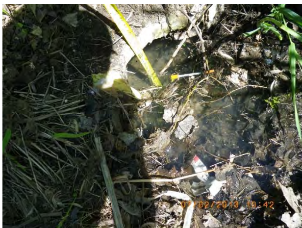
Figure 65 - Severe deposition at outfall 15-1903
