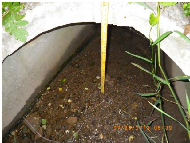
Figure 43 - Minor deposition at outfall 13-1588
