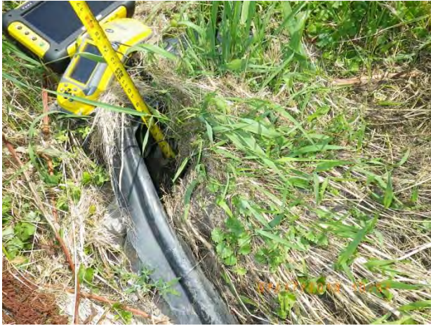
Figure 51 - Severe deposition at outfall 14-1218
