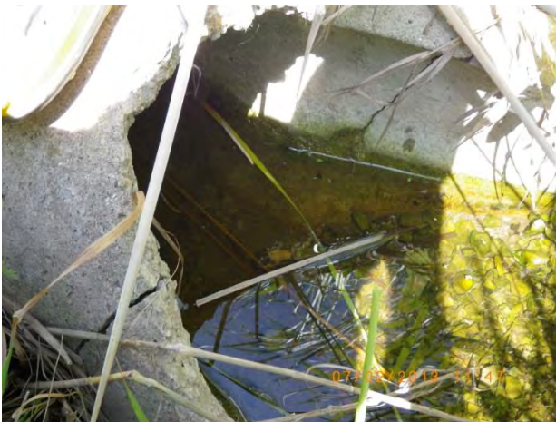
Figure 26 - Crack on apron walls of outfall 12-1916 (minor damage)
