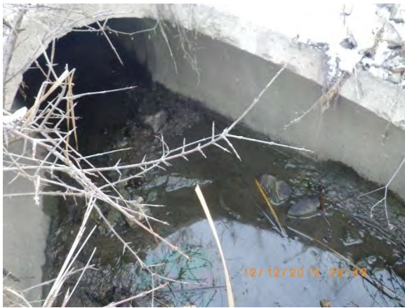
Figure 2 – Oil sheen at the end of the drainage swale
