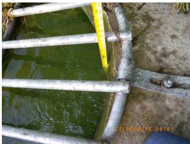
Figure 66 - Moderate deposition at outfall 15-2477
