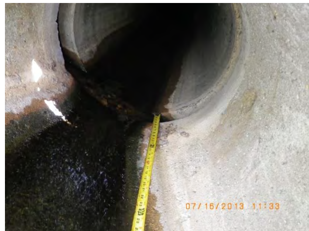
Figure 27 - Outfall 06-1083 apron displacement (minor damage)
