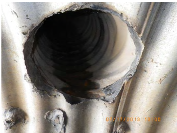
Figure 34 - Outfall 14-675 corrosion (minor damage)
