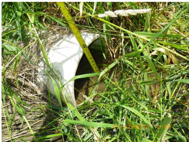
Figure 39 - Moderate deposition at outfall 12-1676a
