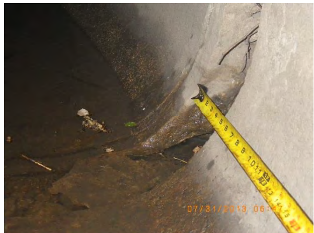
Figure 33 - Outfall 14-660 apron displacement (moderate damage)
