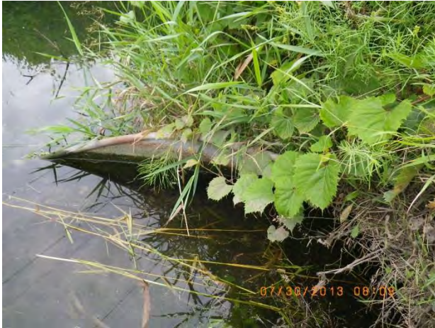
Figure 28 - Outfall 13-1283 corrosion (minor damage)
