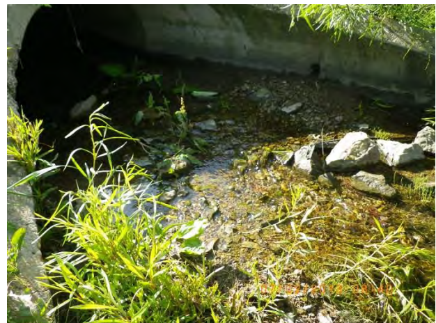
Figure 38 - Minor deposition at outfall 12-1261
