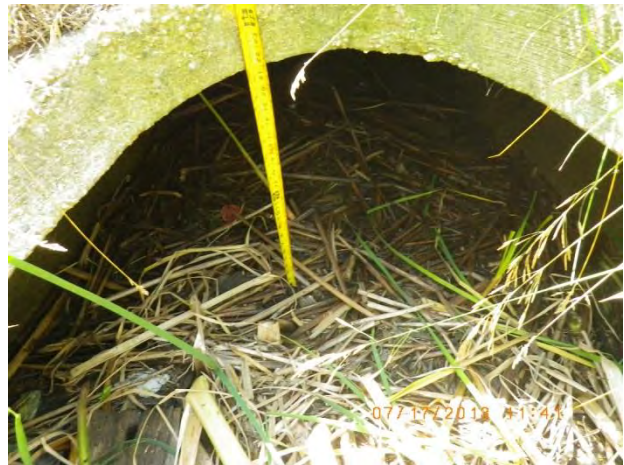
Figure 48 - Minor deposition at outfall 14-1007
