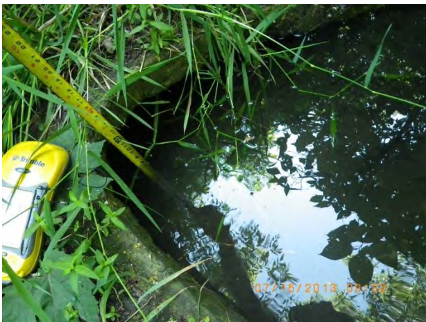
Figure 37 - Moderate deposition at outfall 12-1245
