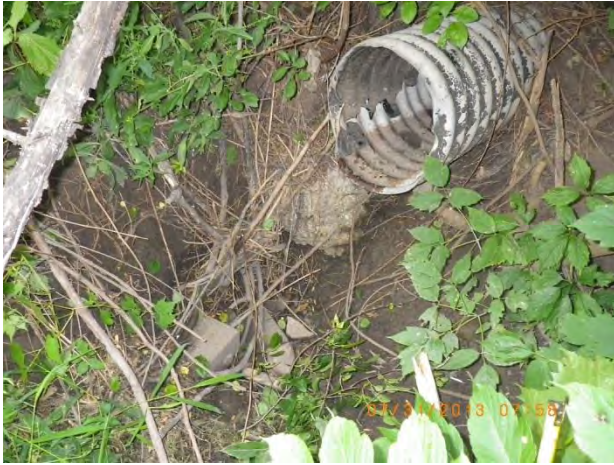
Figure 67 - Minor erosion near outfall 14-124
