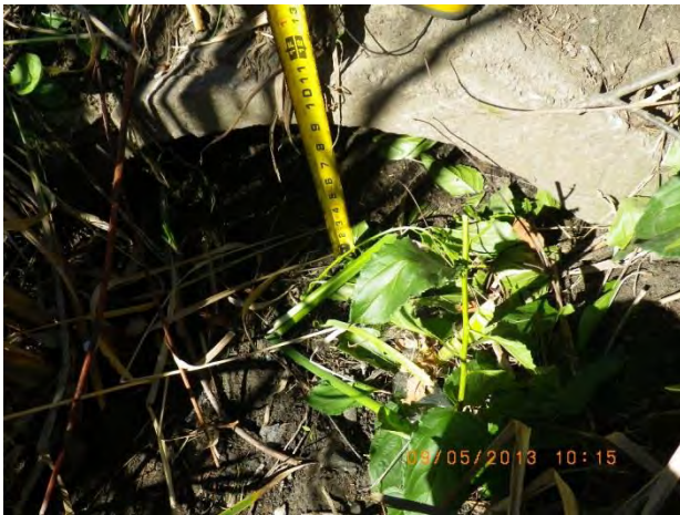
Figure 59 - Severe deposition at outfall 15-1807
