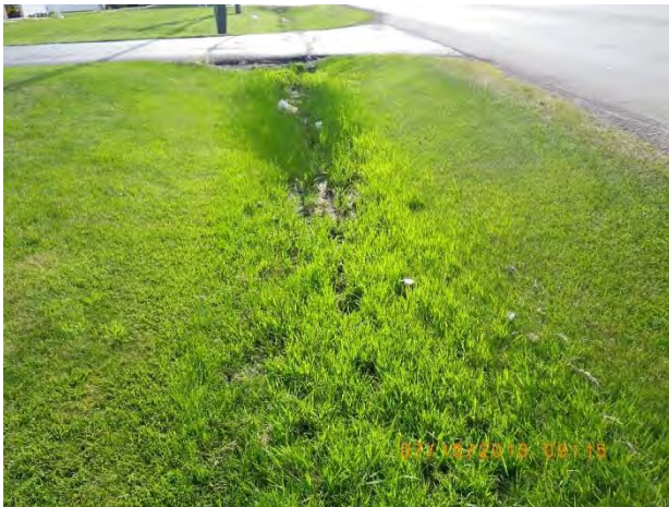
Figure 69 - Minor erosion near outfall 15-1891
