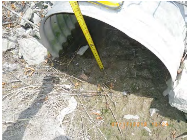
Figure 54 - Moderate deposition at outfall 14-766
