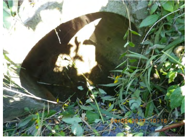
Figure 58 - Minor deposition at outfall 15-1806
