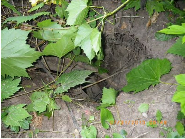
Figure 68 - Moderate erosion (sinkhole above joint) near outfall 14-660
