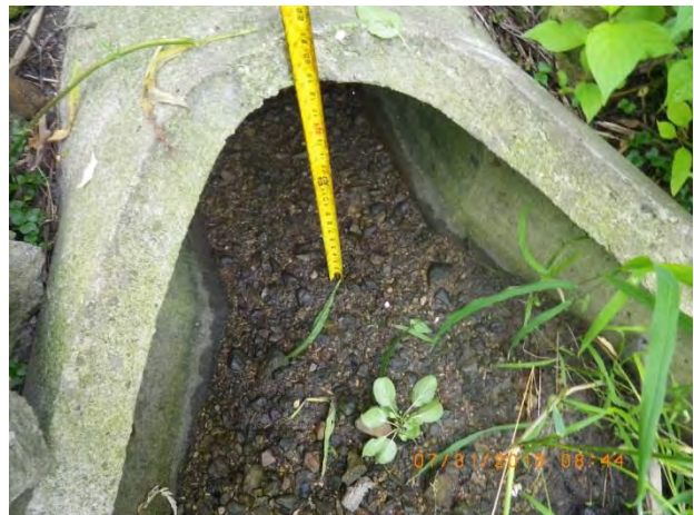
Figure 50 - Minor deposition at outfall 14-1138
