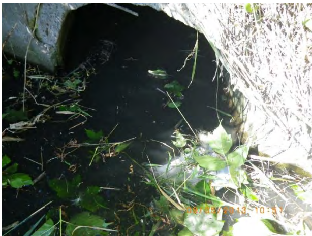
Figure 61 - Moderate deposition at outfall 15-1856
