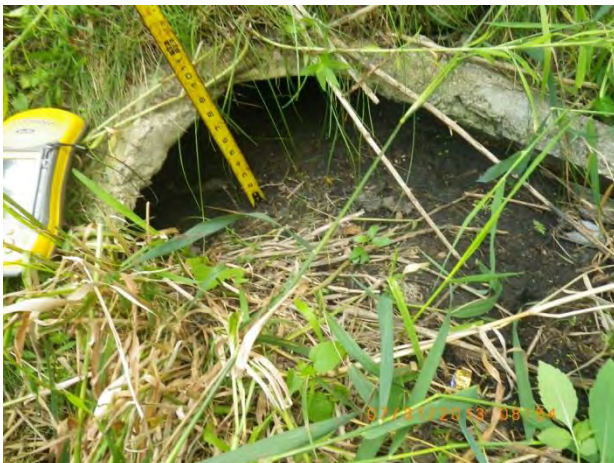
Figure 49 - Severe deposition at outfall 14-1136
