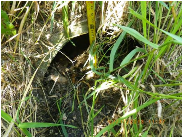
Figure 53 - Moderate deposition at outfall 14-670
