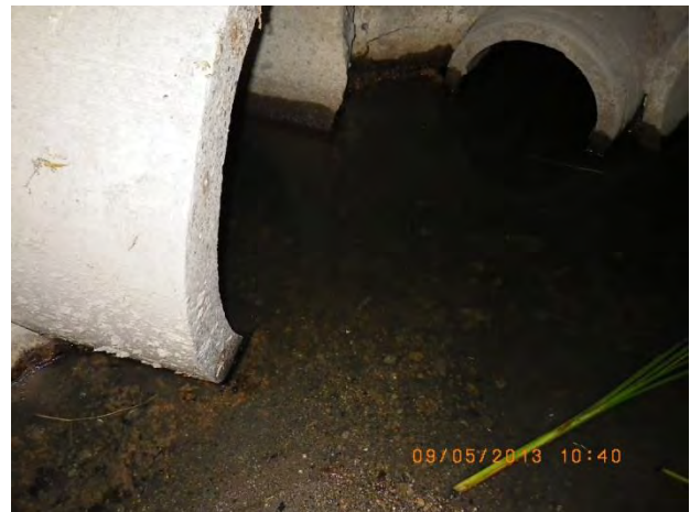
Figure 62 - Minor deposition at manhole 15-1856 US1
