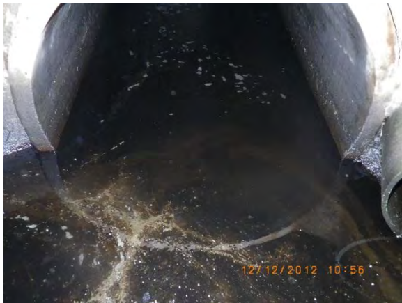
Figure 10 – Drainage swale pipe connection to manhole 13-1743
