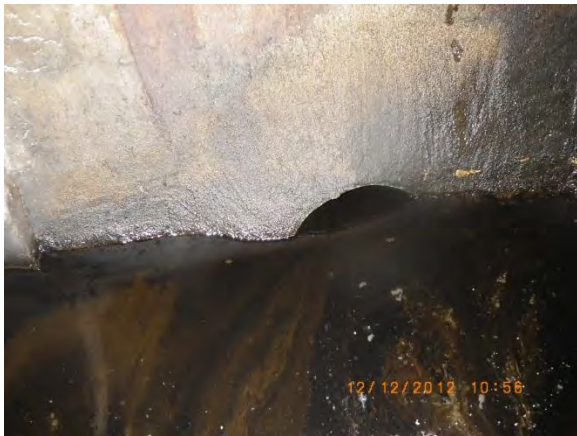
Figure 9 – Detention pond outlet pipe connection to manhole 13-1743
