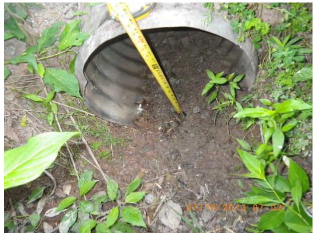
Figure 56 - Minor deposition at outfall 15-1734
