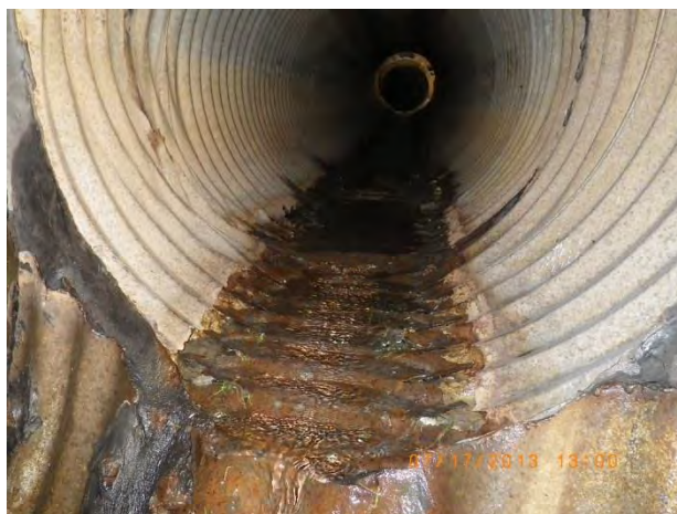
Figure 35 - Outfall 14-676 corrosion (moderate damage)
