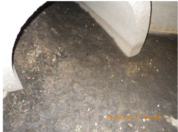
Figure 60 - Moderate deposition at manhole 15-1807 US1
