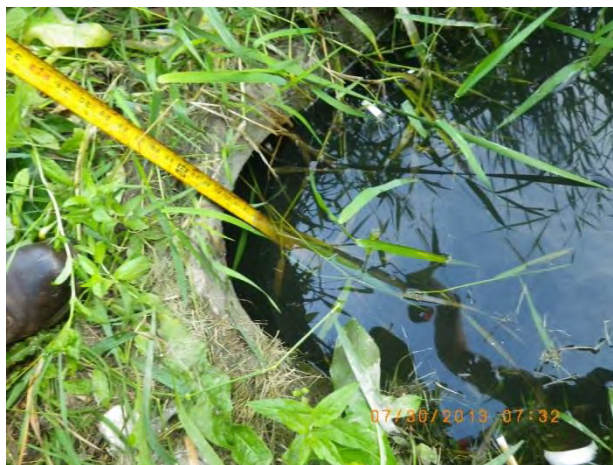
Figure 44 - Moderate deposition at outfall 13-1758
