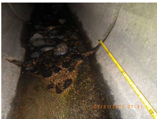
Figure 36 - Outfall 14-999 apron displacement (minor damage)
