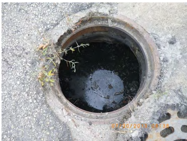
Figure 41 - Minor deposition in manhole 13-1098 US1
