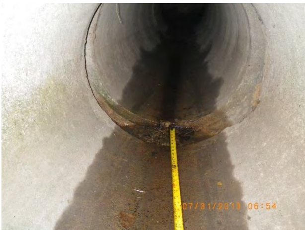
Figure 32 - Outfall 14-659 apron displacement (moderate damage)
