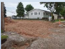
TRACKING PAD NOT INSTALLED
