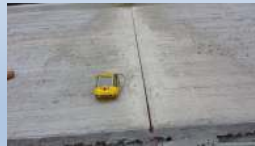
CONCRETE SAW CUTTING AFTER PAVING (WINDROW THAT REQUIRES REMOVAL)
