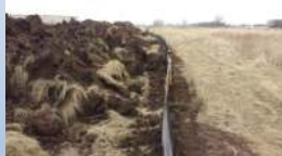
A PROPERLY INSTALLED SILT FENCE WITH COMPACTION
