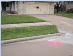
CONCRETE SAW CUTTING BEFORE PAVEMENT REMOVAL (NOT CLEANED UP)
