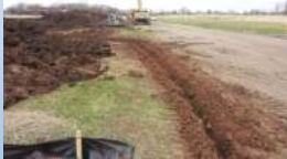
A PROPERLY INSTALLED SILT FENCE TRENCH
