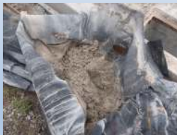
CONCRETE WASHOUT INTO AN INLET PROTECTION (UNAPPROVED)
