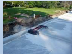
CONCRETE SAW CUTTING WITH INLET PROTECTION INSTALLED AND STONE BAGS
