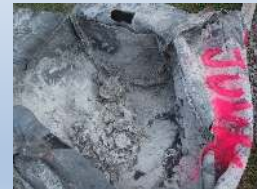
CONCRETE SAW CUTTINGS COLLECTED BY INLET PROTECTION
