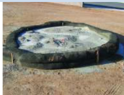
CONCRETE WASHOUT INTO SIMPLE CONTAINMENT AREA (APPROVED)
