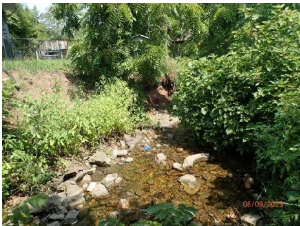
Figure 31 – Channel erosion downstream of outfall 13-471
