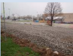
PROPERLY INSTALLED TRACKING PAD
