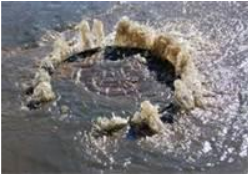
Sanitary Sewer Overflow Occurs
