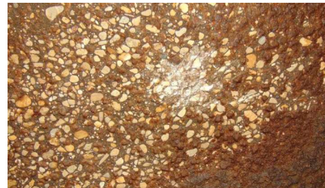
Damaged Concrete Surface
