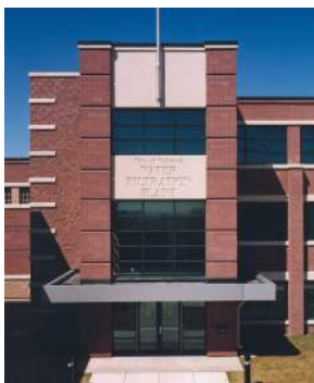
Oshkosh's Water Filtration Plant constructed in 1999
