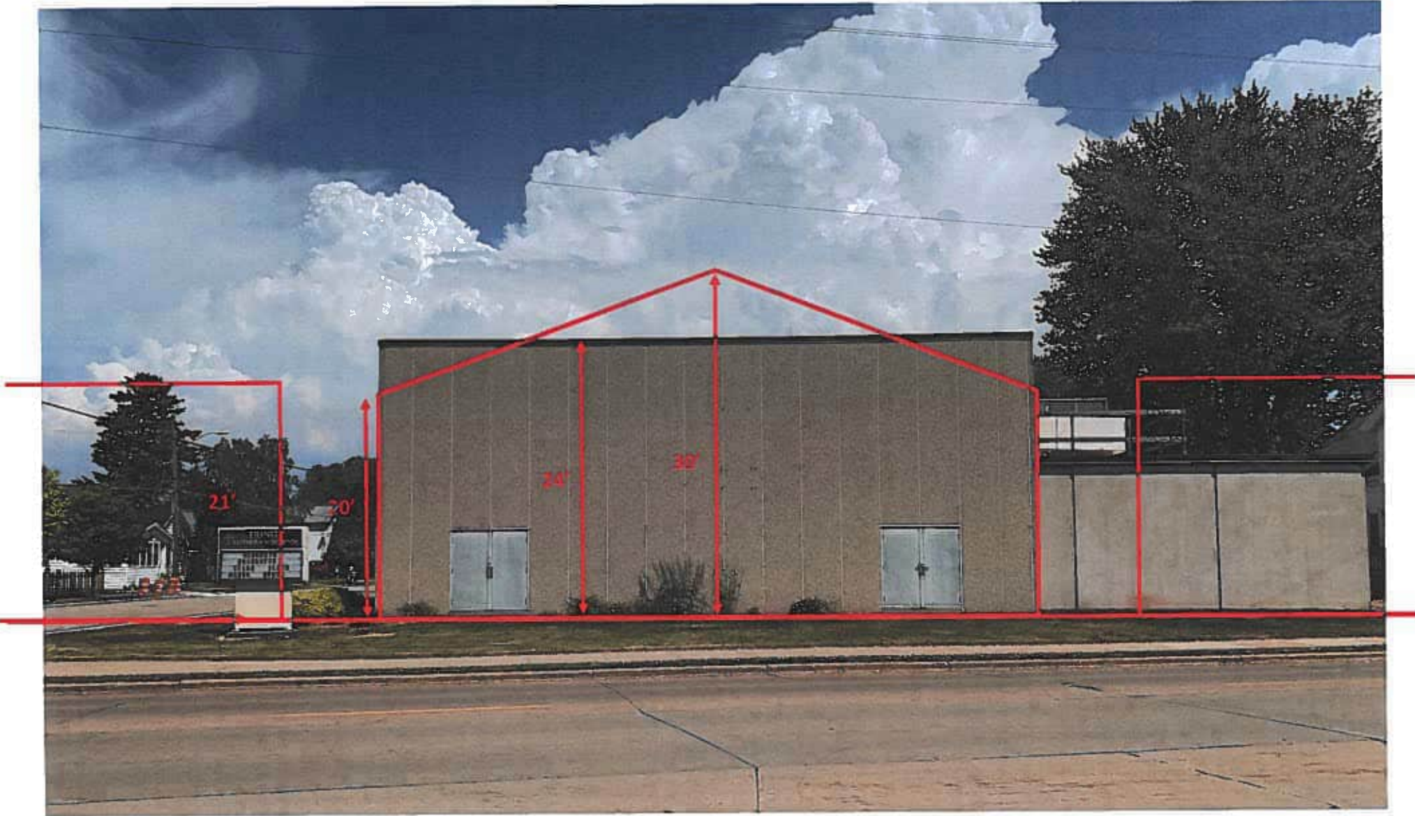
Clearwells and Pump House Size Comparison to Trinity Lutheran Gymnasium on Bowen Street
