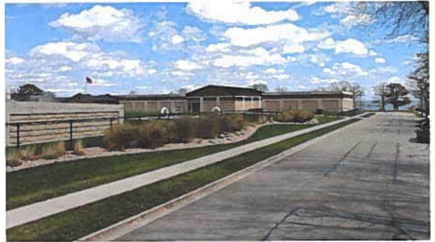
View of Washington Avenue with Clearwells and Pump House
