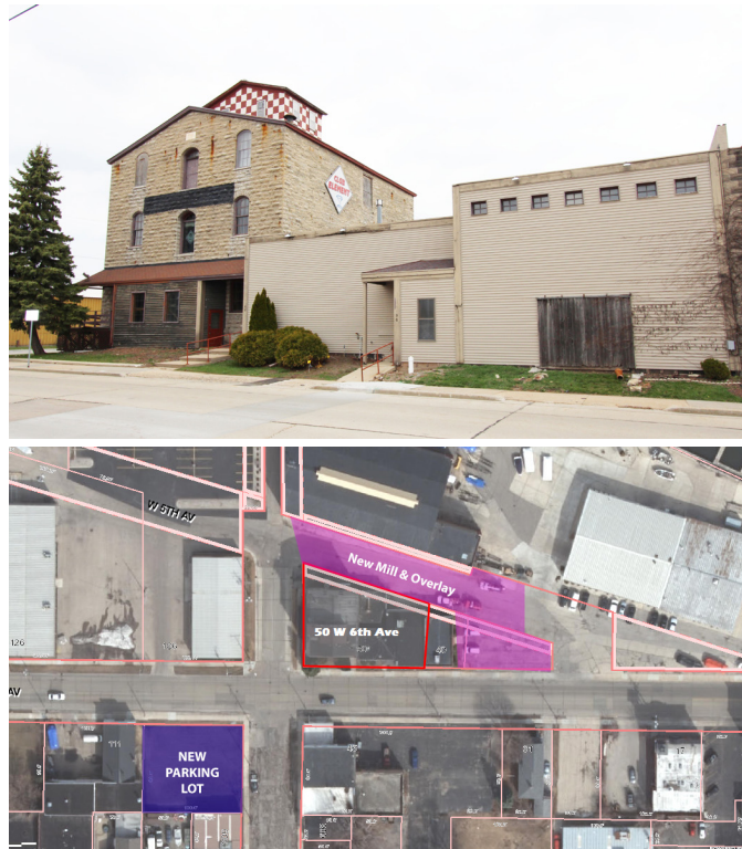
Figure 1 - Front elevation and overhead view of site
