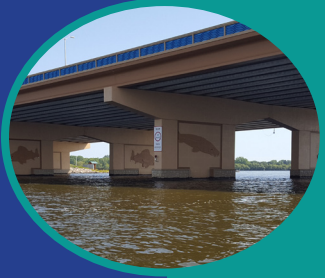
21 TRIBAL HERITAGE CROSSING BRIDGE
