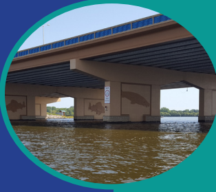
21 TRIBAL HERITAGE CROSSING BRIDGE
