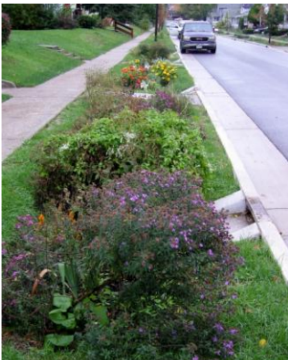
Fig 2. Bioretention incorporated into a right-of-way. This can be incorporated either on streets leading towards main
