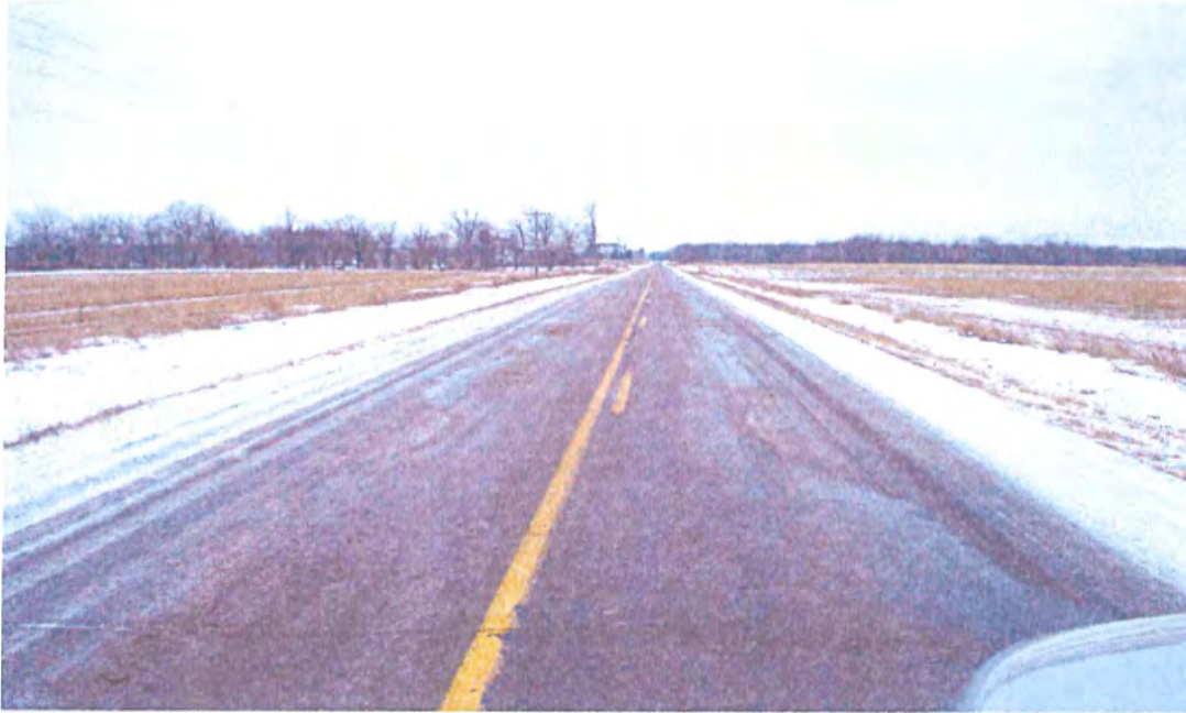
CTH D 2-12-09 400lbs per lane mile with 30% salt sand with Salt Brine
