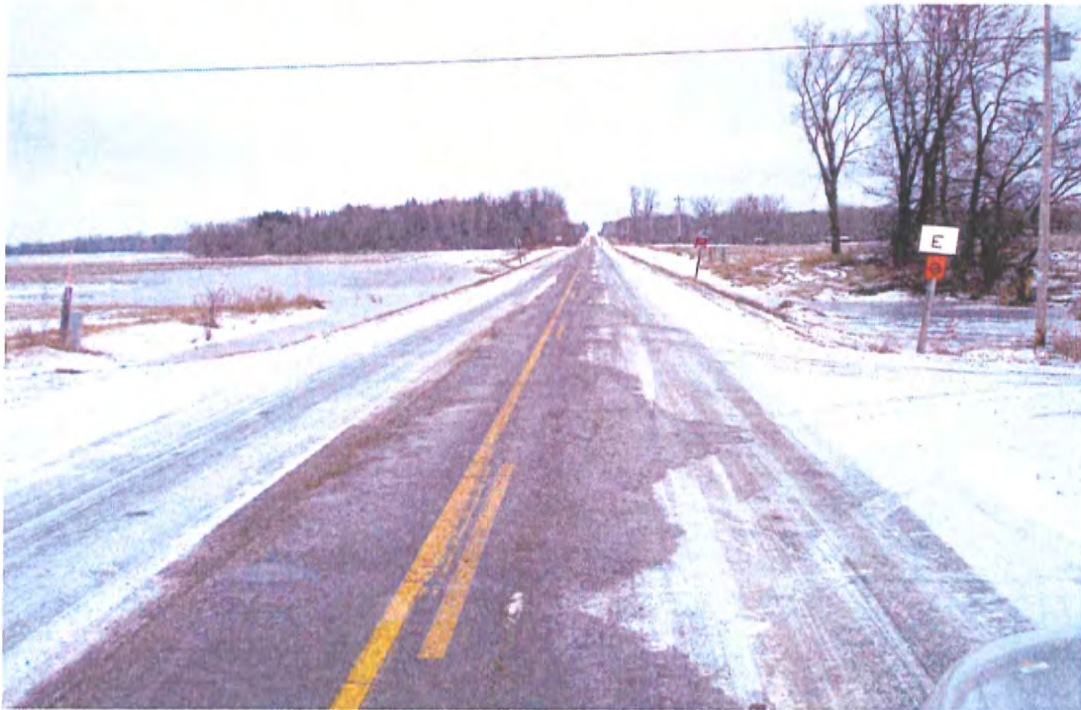
CTH E 2-12-09 600lbs per lane mile with 30% salt sand with out Salt Brine
