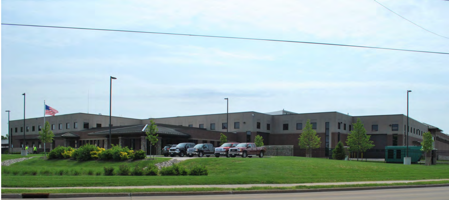
Oshkosh Facilities Maintenance Building - courtesy of Sue Panek
