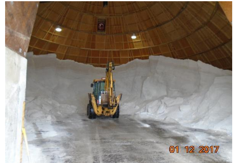
Salt shed at Field Operations Facility
