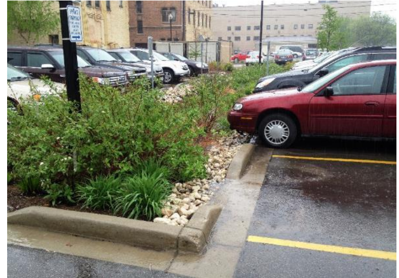
400 North Main Street Parking Lot Biofilter
