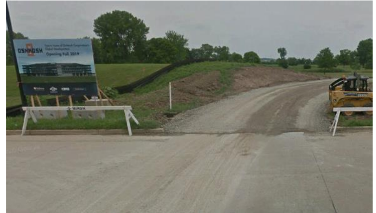
Oshkosh Corporation Headquarters Construction Entrance
