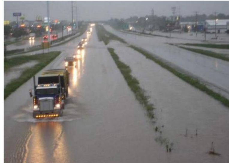
Highway 41 flooding during June 12, 2008 storm event
