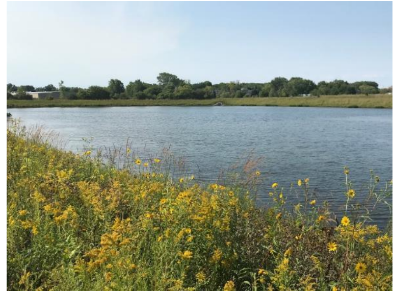
Fernau Watershed - North Main Street Wet Detention Basin
