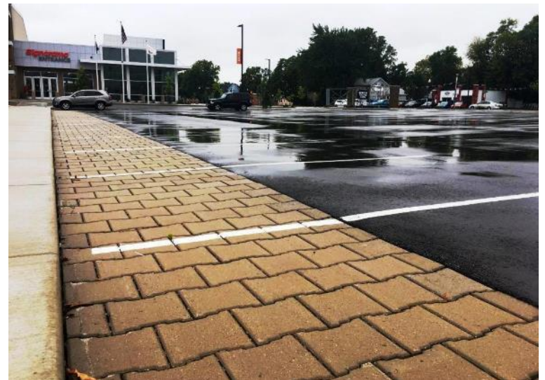
Menominee Nation Arena Porous Pavement
