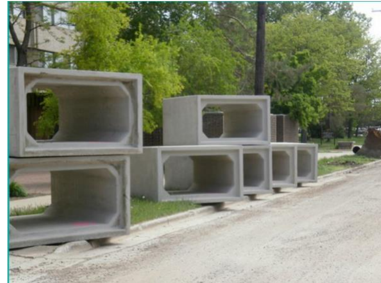
Box culvert installed as part of street reconstruction project
