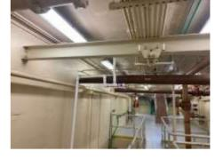
This project will replace the lifting beam that is located above the blended sludge pit, and add a davit crane in the headworks for equipment removal.
