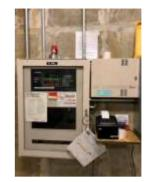
Replace fire alarm system installed in 1994: Simplex/Grinnell 4020 Upgrade to 4100U (or equivalent) Addressable Controller and replacement of all initiating devices (smoke detectors, ductwork smoke detectors, and heat detectors) except pull stations.
