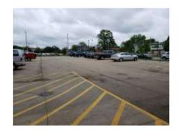
Station 15. 101 Court St. - Asphalt parking lot surface is deteriorating and requires crack filling and slurry seal coat. According to the May 2020 Assessment of Municipal Parking Lots report by Jewell Associates Engineer for the City of Oshkosh, Station 15 should be considered for spot improvement & slurry seal. Refer to Exhibits 8.1, 8.2 and 8.3 of the Report
