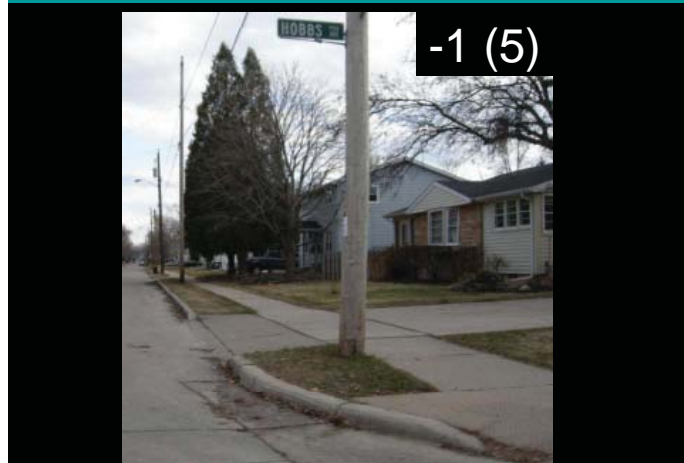
Line 24 Residential sidewalk with narrow Terrace
