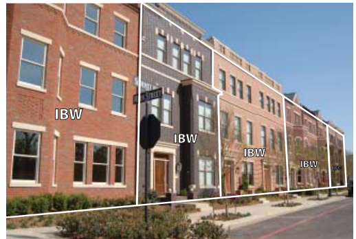
An Individual Building Width (IBW) is the division of a façade into distinct modules or sections. Although sections of a single façade share a common design vocabulary, each section should be distinguishable from its adjacent modules. IBWs can be distinguished by changes in material, color, window and door treatment, masonry pattern, cornice treatment or appropriate combinations of these items.
