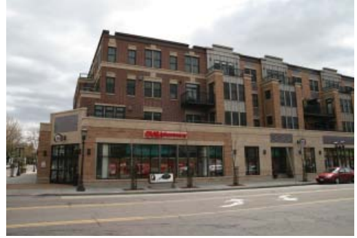
This mixed-use building with retail on the ground floor and housing above utilizes a series of building setbacks to maintain a comfortable pedestrian realm and create architectural interest.
