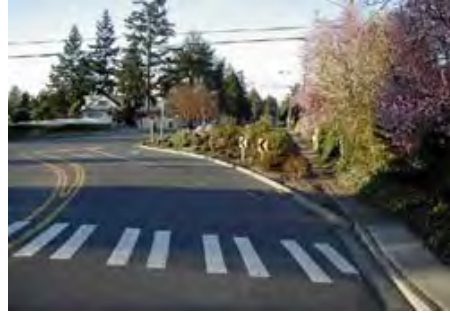
This skewed intersection was modified to slow vehicle speeds and increase awareness at the intersection.
