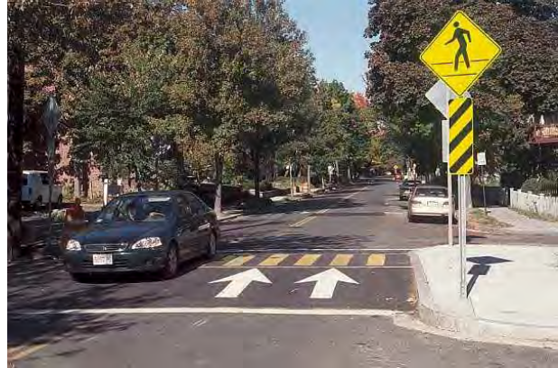
Engineering Improvement – Bulb-out, crosswalk, pedestrian sign & speed bump
