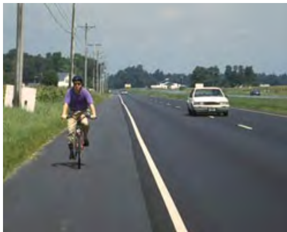
Photograph depicting a paved shoulder
