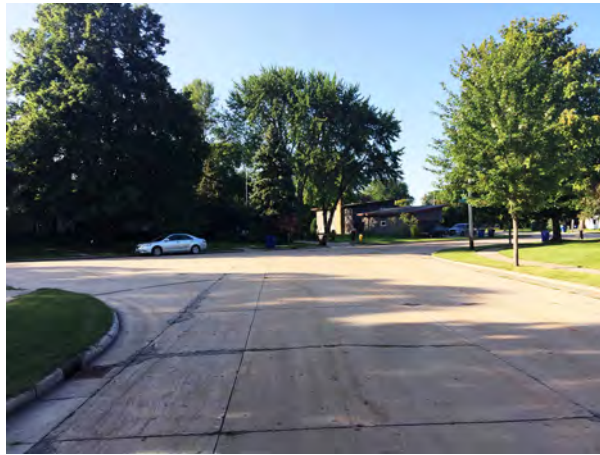
Large and uncontrolled intersection on White Swan Drive
