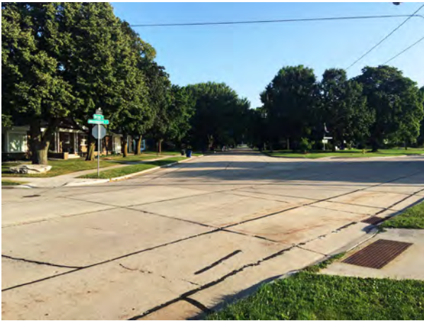
Oversized intersection along Menominee Drive
