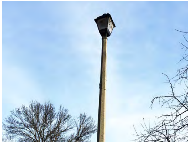
Concrete light pole with ornamental fixture
