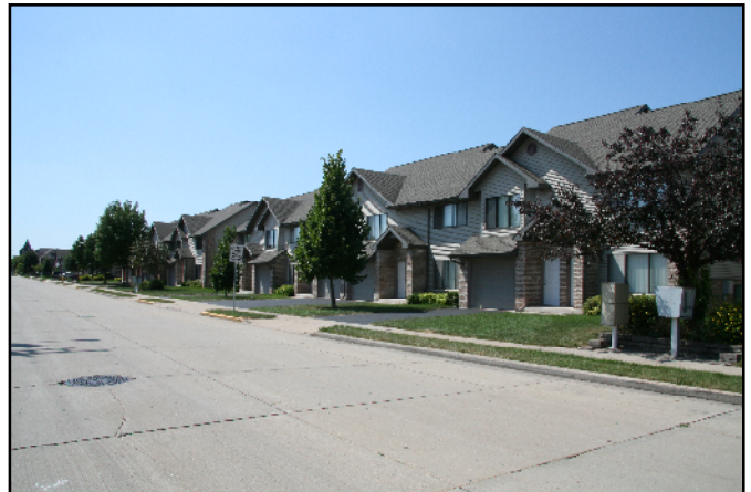
Burns Townhome Development - located on Division Street between W. Irving Avenue and Church Avenue.
