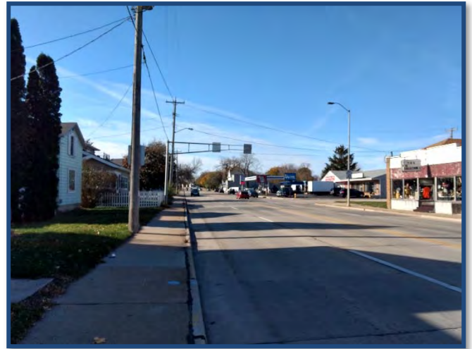
Oshkosh Ave (STH 21) just west of N. Sawyer St - looking west
